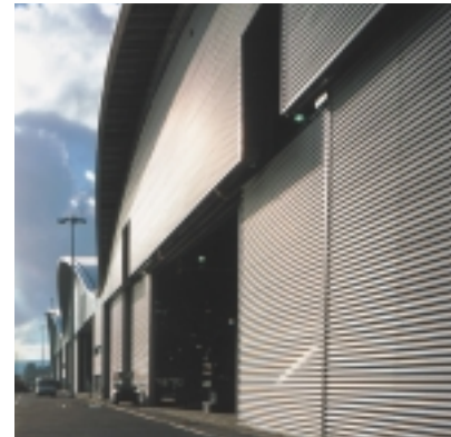
New Hangars for TAG Farnborough Airport - Rowecord Engineering Ltd
