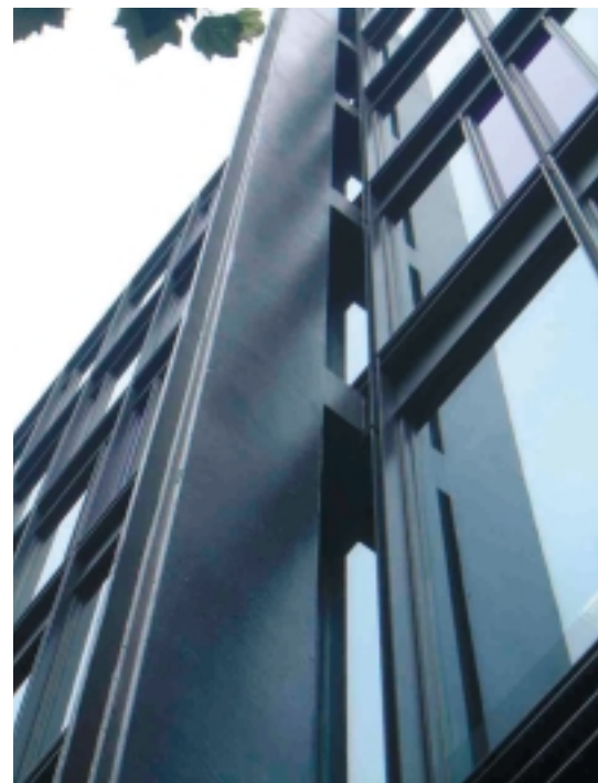
Mid City Place, Holborn with fabricated external box columns with rigid box beam spigots through the cladding spliced internally to floor beam.
