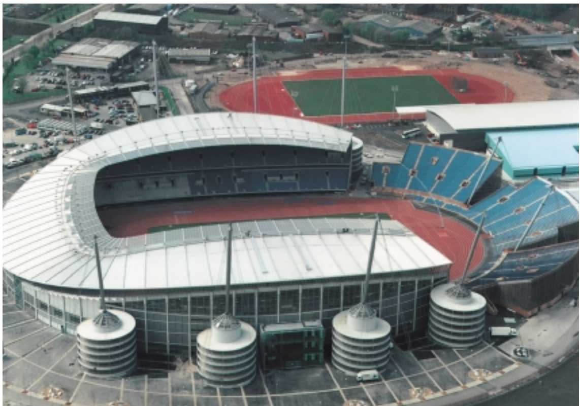
City of Manchester Stadium - Watson Steel Structures Ltd
