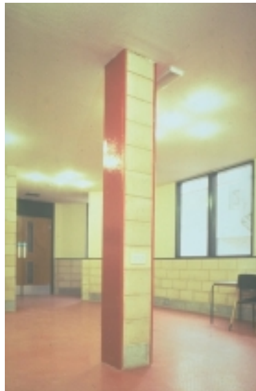
Block-filled column providing 30 minutes fire resistance
