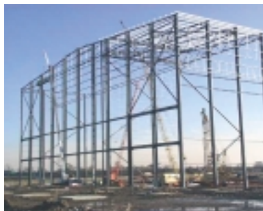
High bay, large span lattice girder roof
