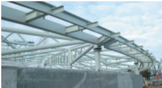
Water Treatment Works, Lowestoft - Westbury Structures Ltd
