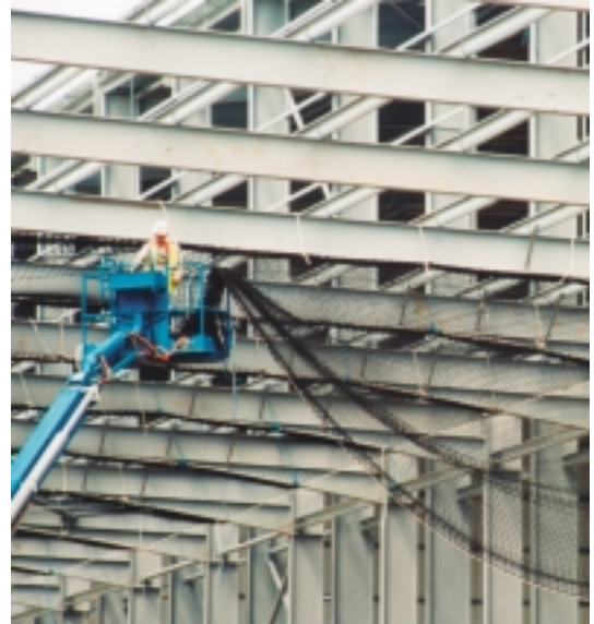
Ikea, Peterborough – Billington Structures Ltd
