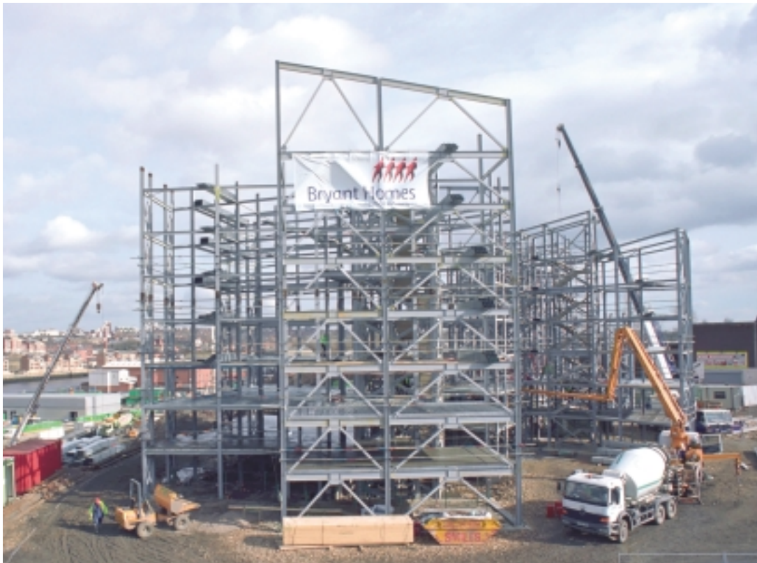
Baltic Quays Residential Block, Gateshead – Severfield-Reeve Structures Ltd
