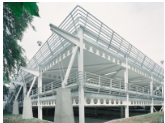
Car Park, Amersham – Conder Structures Ltd
