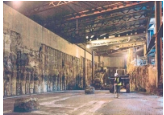
Sub-basement blinded, piles to be trimmed for stanchions to support first basement perimeter bays yet to be built.
