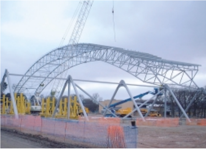
Category H Steelwork - TAG Aviation Hangar, Farnborough – Rowecord Engineering Ltd
