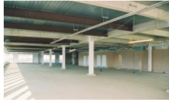
Project "Time" showing unprotected secondary beams in composite metal deck construction
