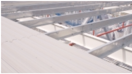
Roof Decking, Airbus (UK) Ltd, Broughton – Corus Panels & Profiles
