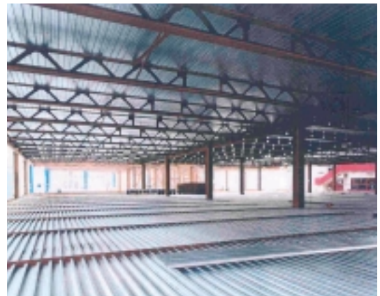
5th Floor decking laid prior to concreting (3rd concreted).
