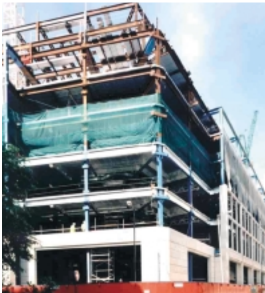
Deck bundles delivered to 6th; 5th floor decked; 3rd concreted. Cladding to 3rd floor.
