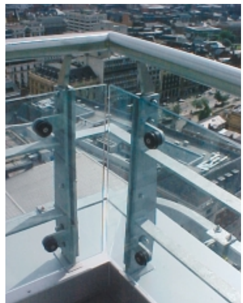
Category L Steelwork - Terrace Balustrading – Glentworth Fabrications Ltd
