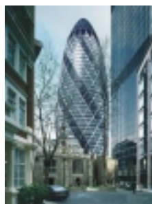
Swiss Re Building. Fire Engineers Arup Fire.
