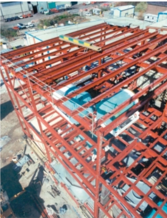
Category C Steelwork - Volclay, Wallasey - Henry Smith (Constructional Engineers) Ltd
