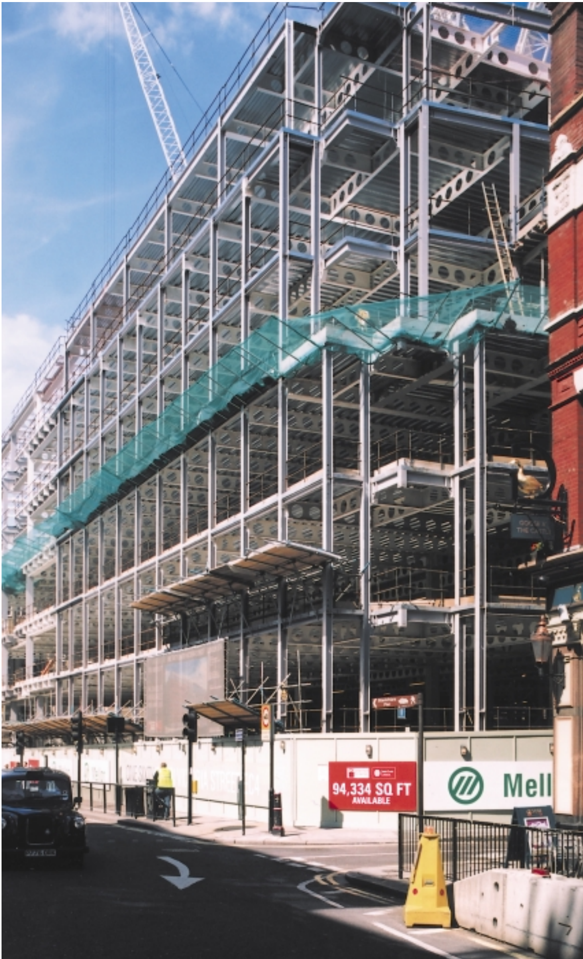
Category D Steelwork - Times Square, London – William Hare Ltd
