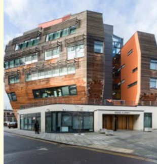
Bridge Academy Hackney
