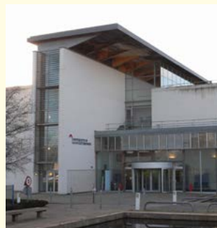
Oxtalls Campus, University of Gloucestershire
