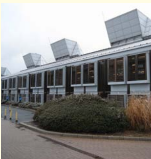
Arup Campus, Blythe Valley Park, Solihull
