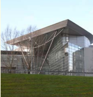
Met Office Headquarters, Exeter
