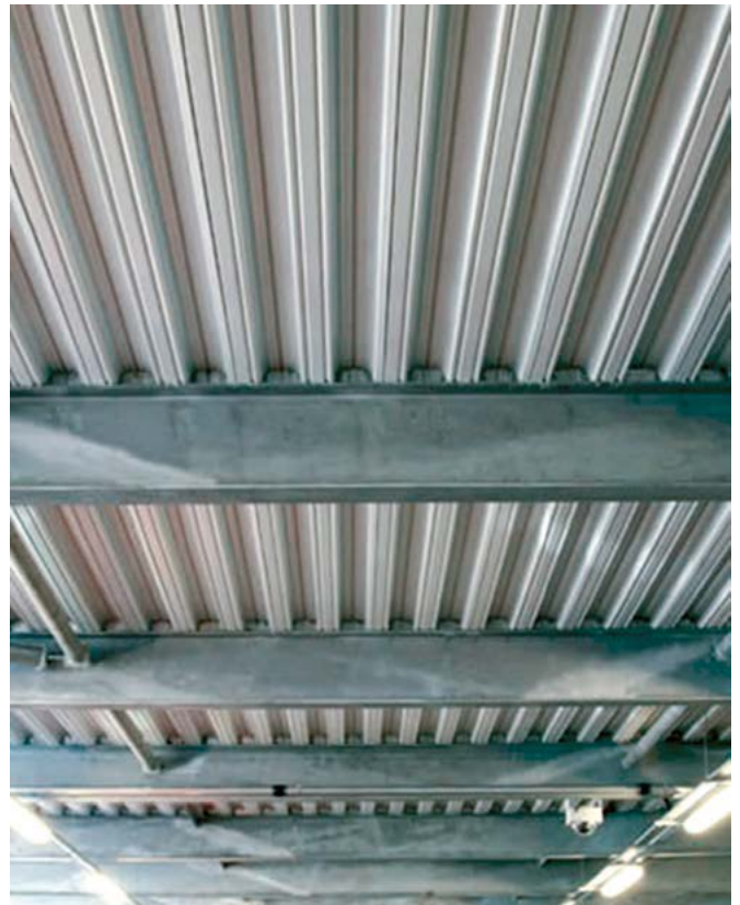
An exposed coated composite steel deck (ComFlor® with Colorcoat FD™25).
