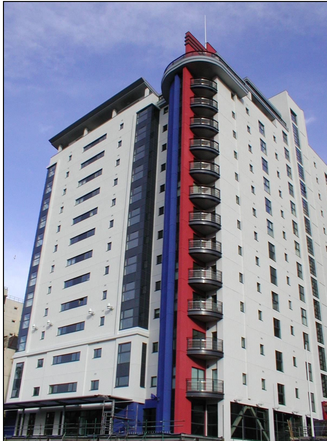
Figure 1.5 Insulated render cladding on light steel framing and a primary steel frame at Landmark Place, Cardiff
