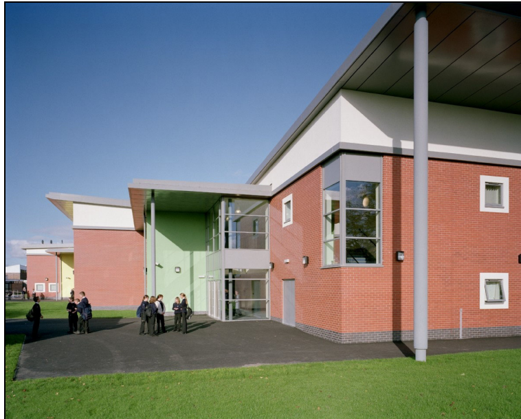
Figure 3.3 Mixed use of brickwork and insulated render in a school building
