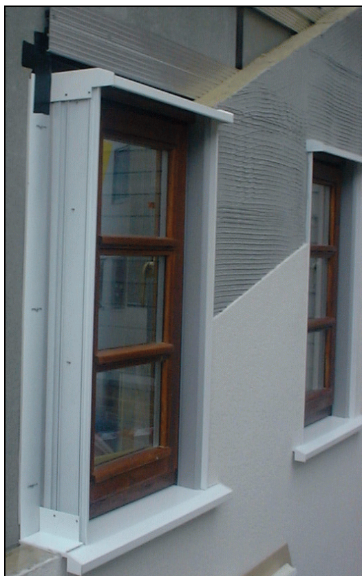
Figure 3.2 Window pod detail and wall build-up
