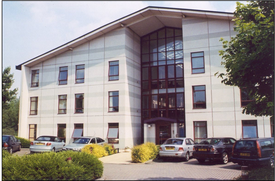
Figure B.2 Belasis Hall, Teesside in its current condition after 16 years
