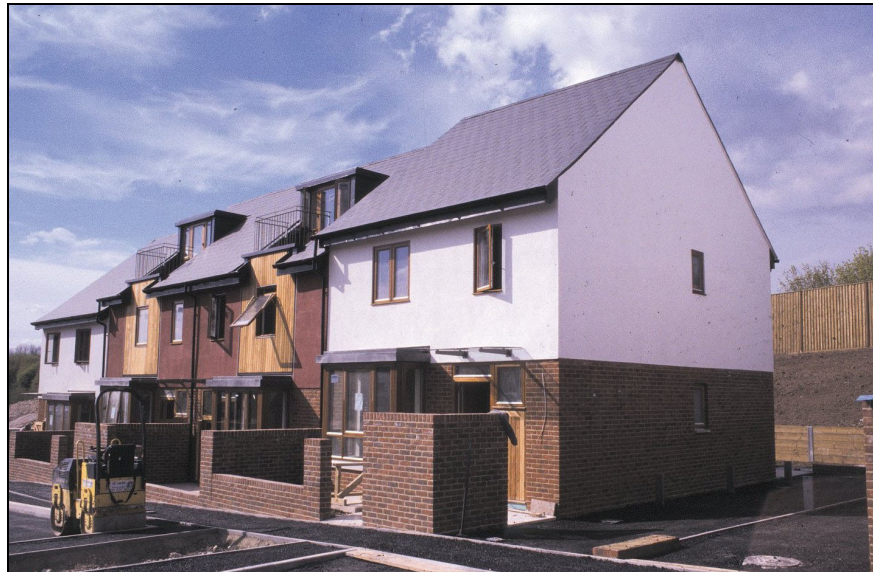
Figure 1.1 Insulated render and brickwork cladding on light steel framed housing, Basingstoke
