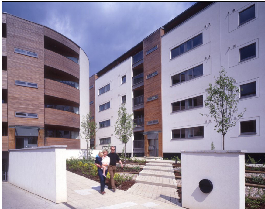
Figure 1.6 Mixed use of insulated render cladding with timber cladding (courtesy of Feilden Clegg Bradley)
