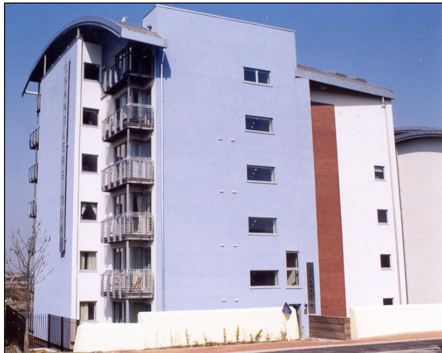
Figure 1.4 Insulated render on light steel infill walls in a composite framed residential building, Penarth Marina, Cardiff
