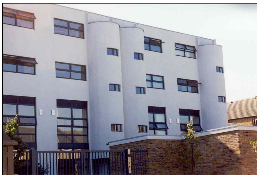
Figure 1.2 Insulated render on light steel framing for an apartment building, Fulham
