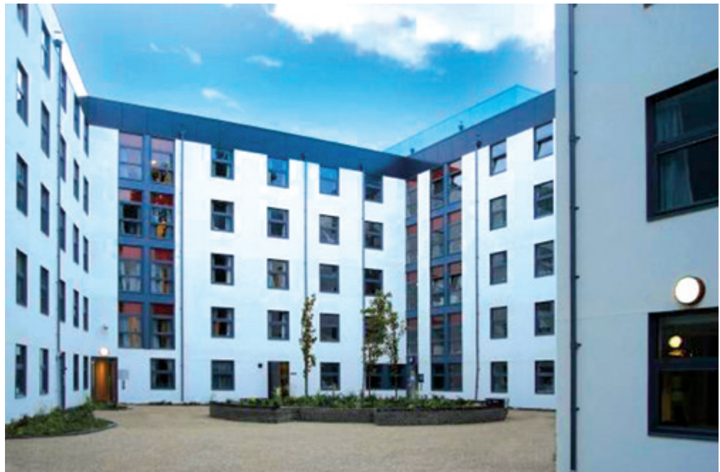
Figure 1.3 Medium-rise accommodation building using light steel framing (Photo courtesy of Fusion Building Systems)
