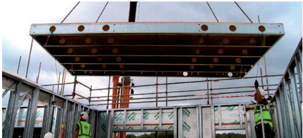
Figure 1.5 Pre-fabricated cassette flooring supported on light steel walls
