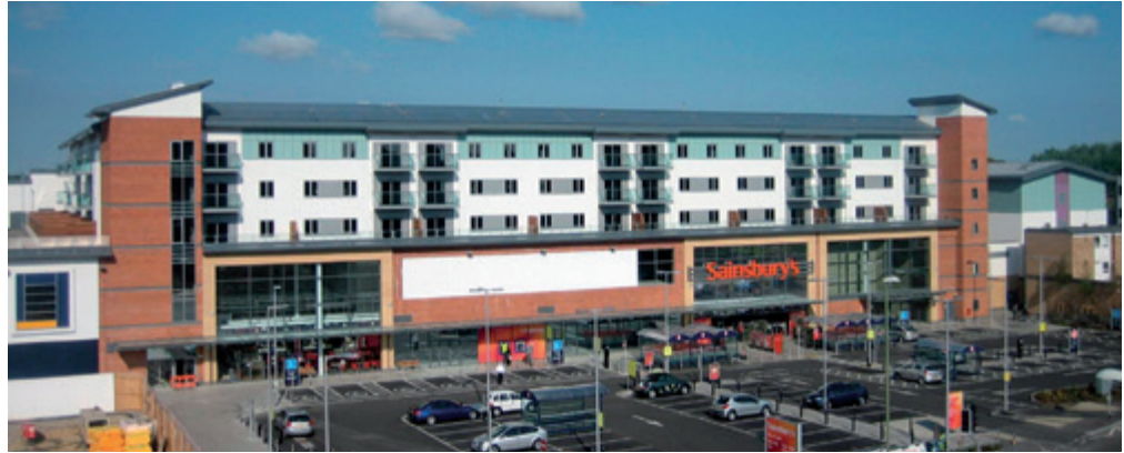
Figure 1.2 Housing using light steel framing built over a supermarket (Photo courtesy of Metek UK Ltd.)
