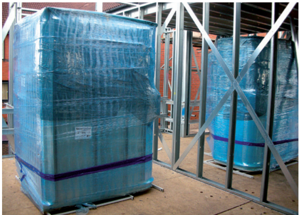
Figure 1.6 Pre-fabricated bathroom pods combined with light steel framing
