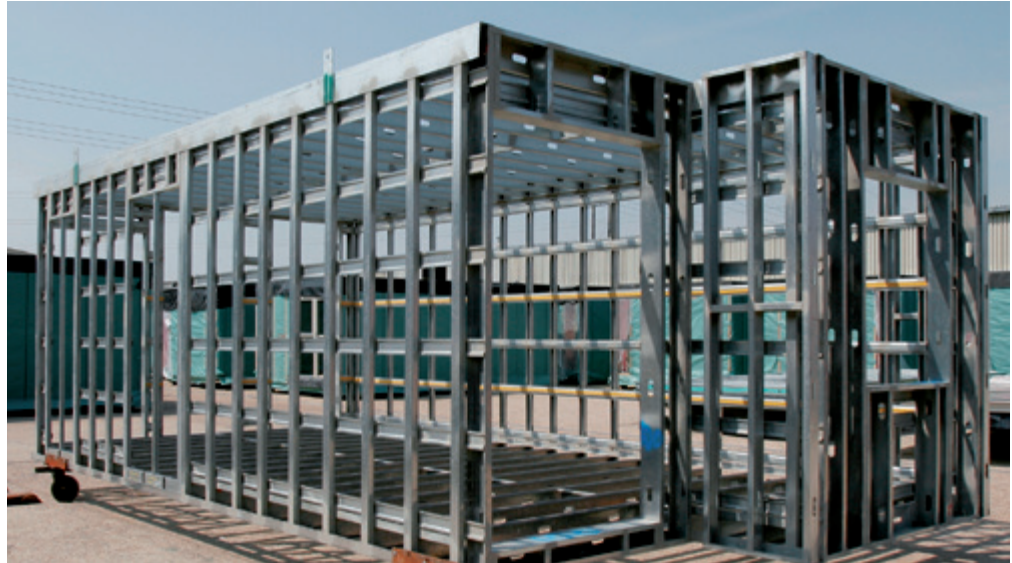
Figure 1.7 Modular construction using light steel framing (Photo courtesy of Ayrshire Framing)
