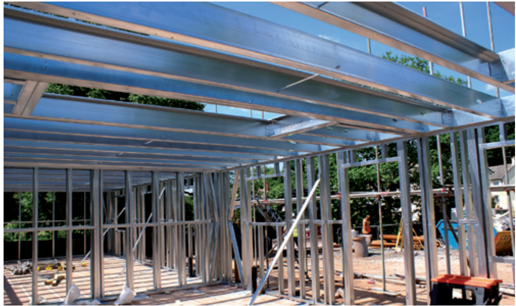
Figure 1.4 Light steel framing using pre-fabricated panels
