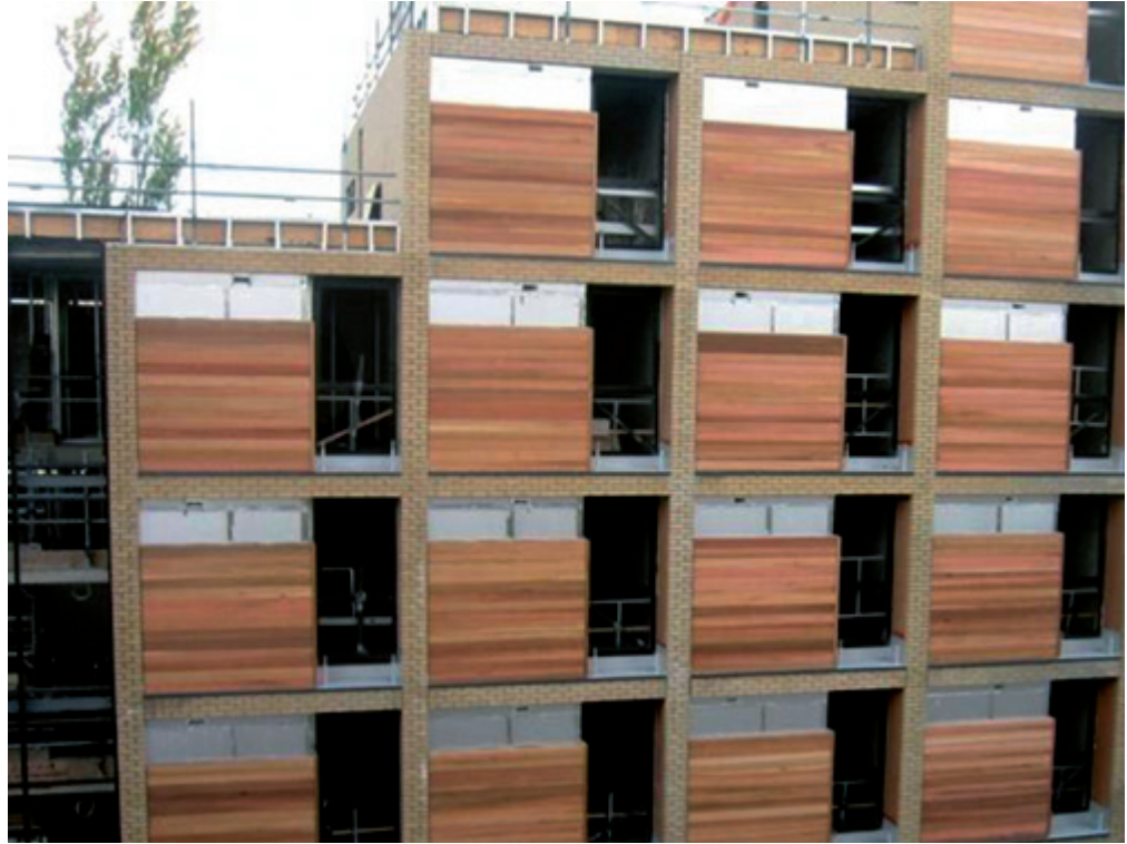
Figure 10.4 Cedar cladding on light steel infill walling (Image courtesy of Metek Building Systems)
