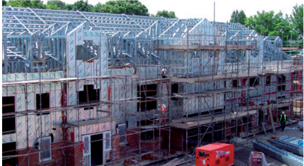
Figure 2.8 Insulated board attached to light steel framework
