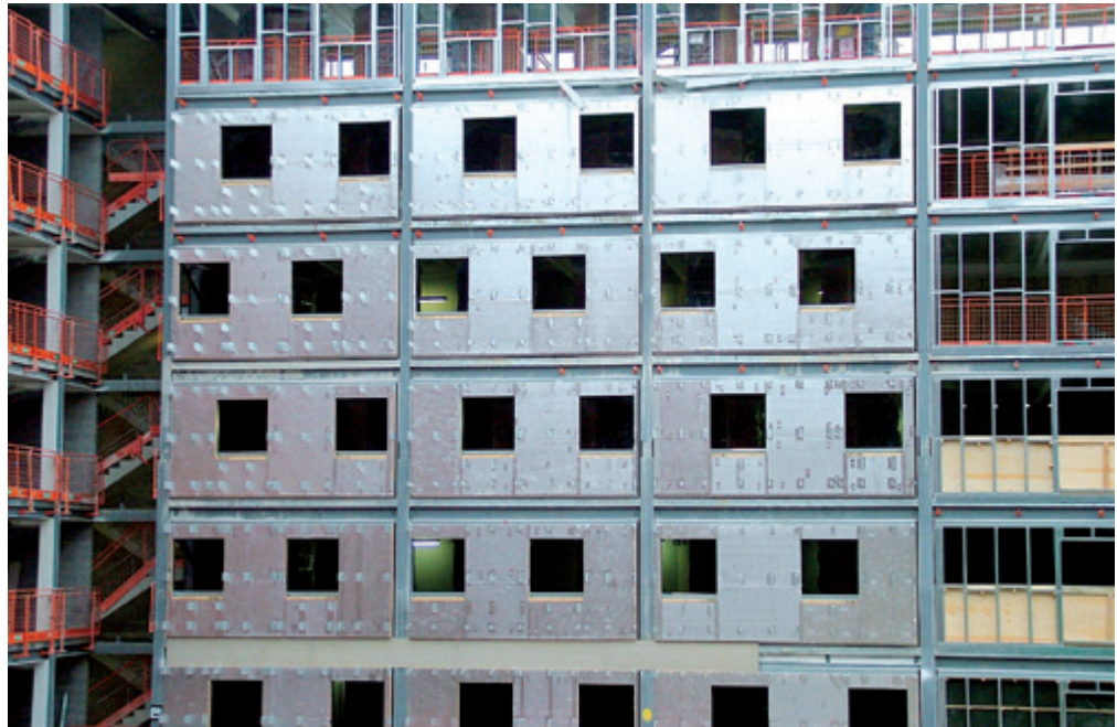
Figure 10.3 Typical prefabricated panelised external wall system
