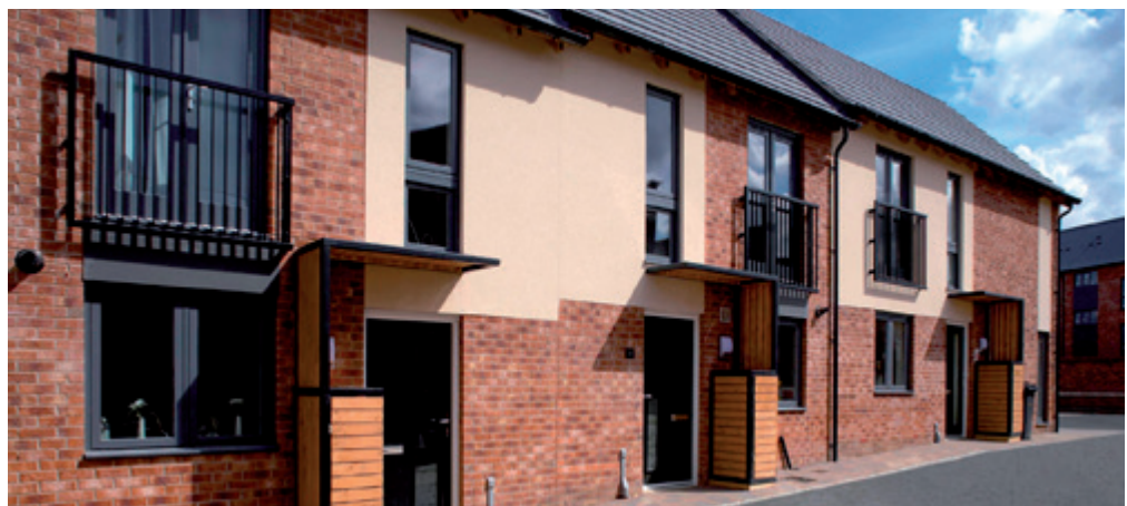
Figure 1.1 Housing using light steel framing
