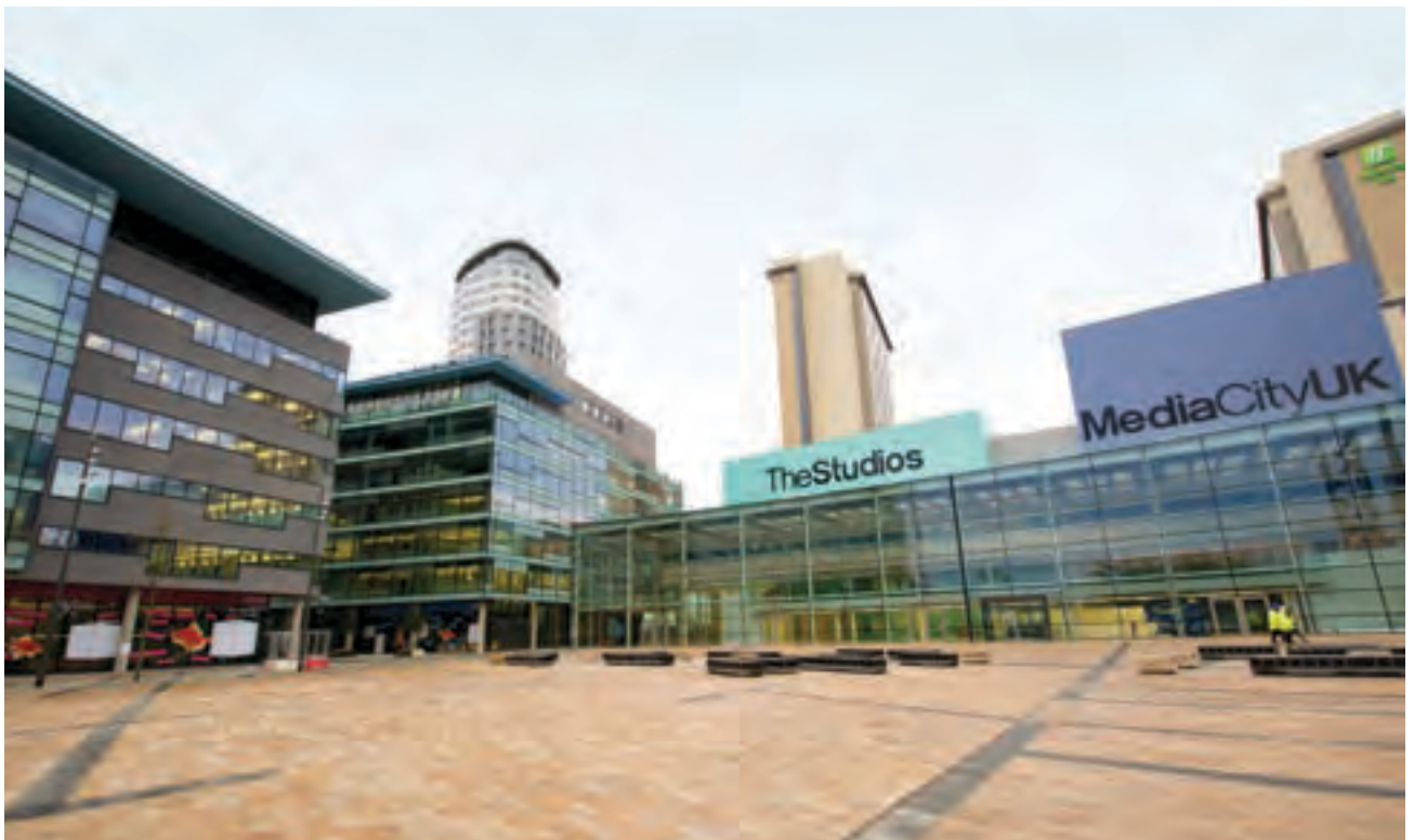
MediaCityUK MAIN STUDIO BLOCK WITH THE ATTACHED HOLIDAY INN TOWER BLOCK
