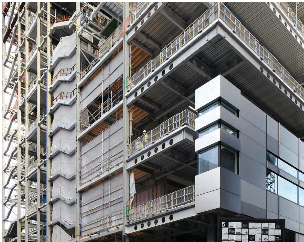
Right Stainless steel cladding was chosen over aluminium to achieve panels that were as flat as possible.
