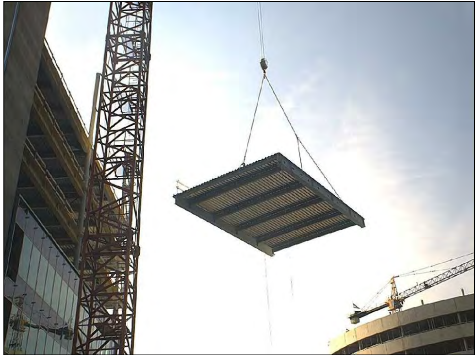
Figure 3.9 Prefabricated floor cassette system
