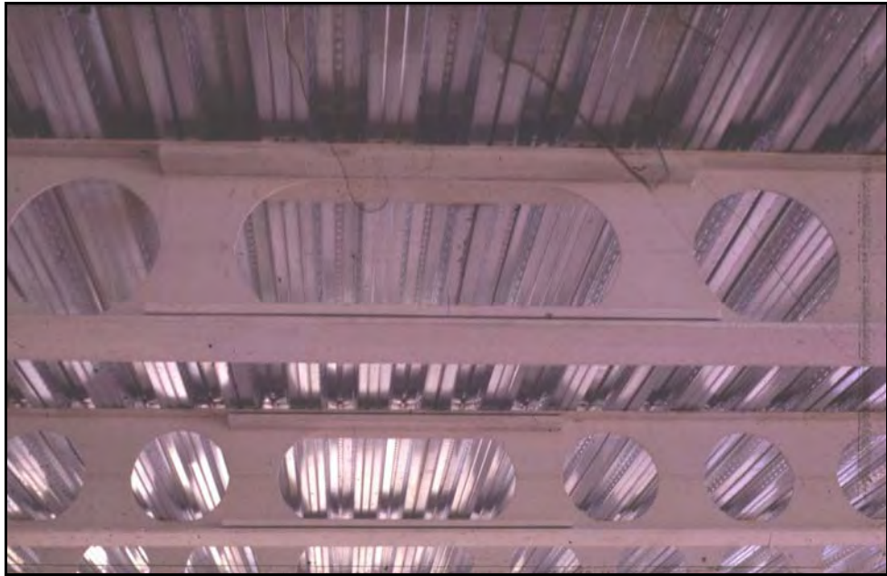
Figure 4.13 Elongated openings with horizontal stiffeners
