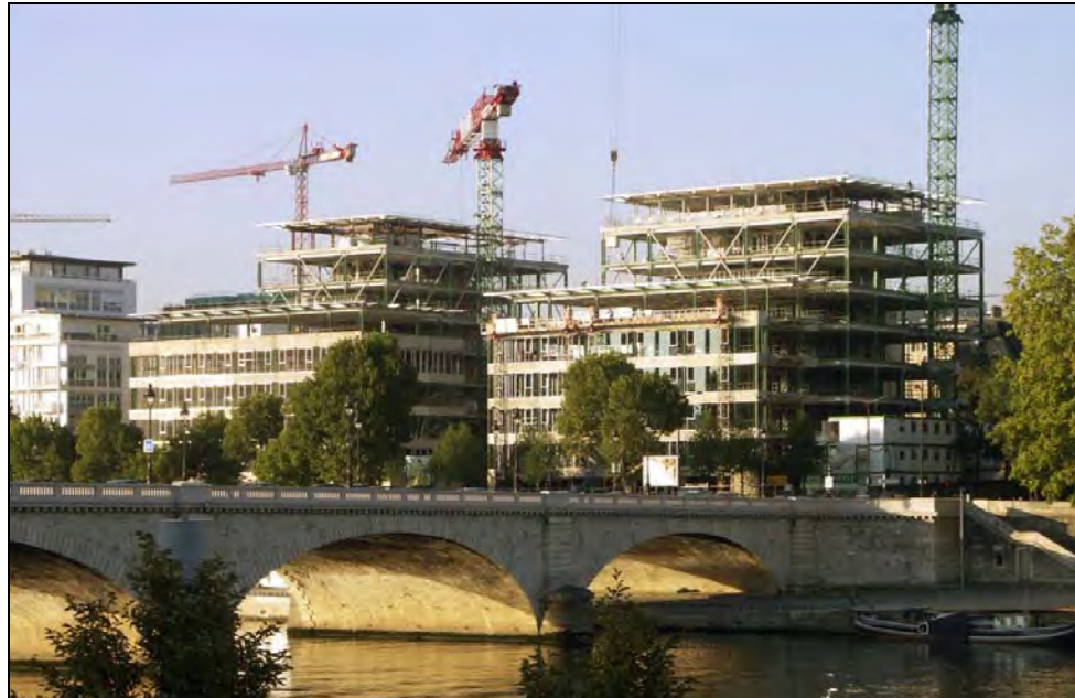
Figure 3.3 Le Seguana buildings, Paris, during construction
