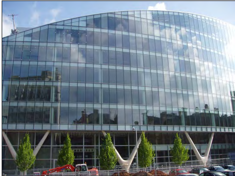
Figure 6.4 Triple glazed wall in a multi-storey commercial building
