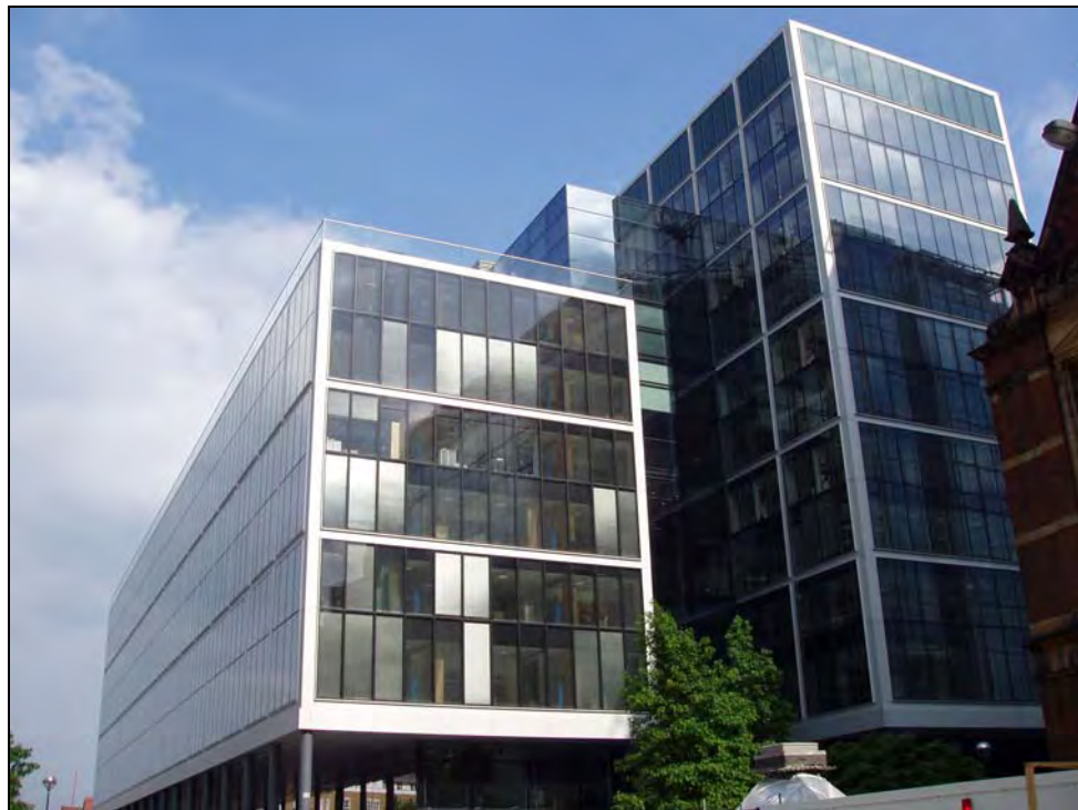
Figure 3.1 Office building, Bishop's Square, London
