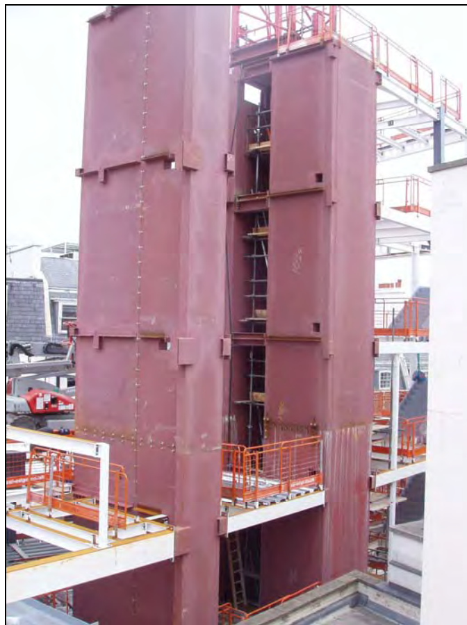
Figure 4.4 Steel composite core speeds up the construction process
