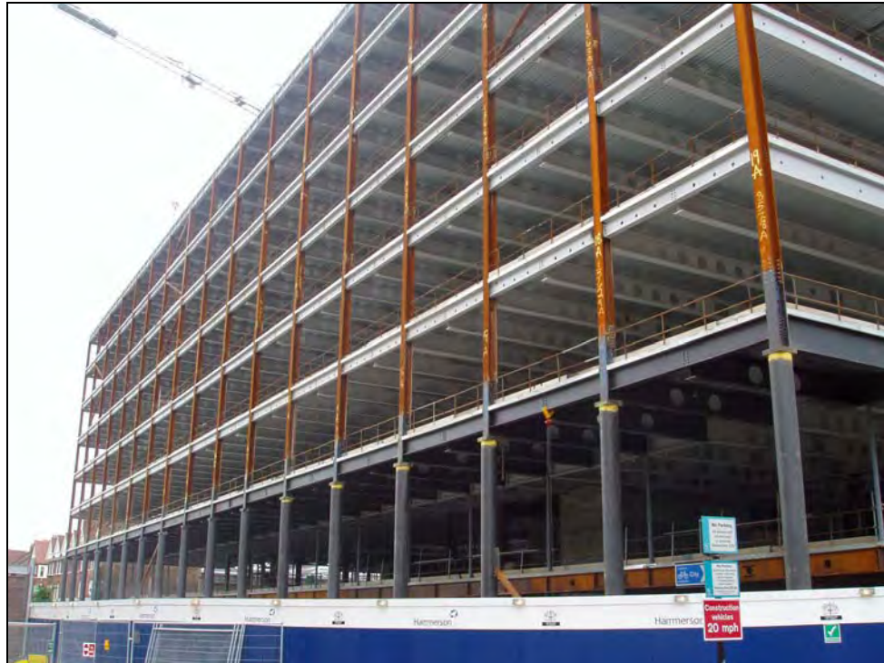
Figure 3.2 View of long span cellular beams in the Bishop's Square project
