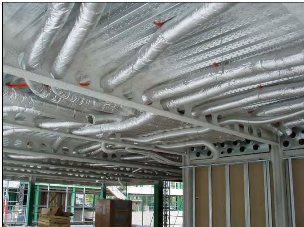
Figure 4.12 Cellular beam with multiple service ducts
