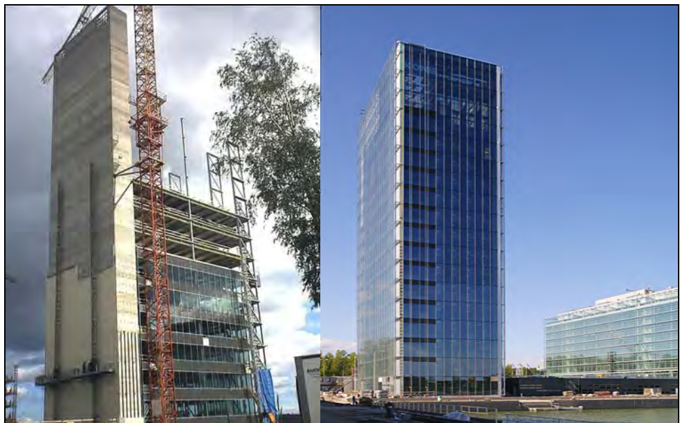
Figure 3.8 Kone building during construction and completed
