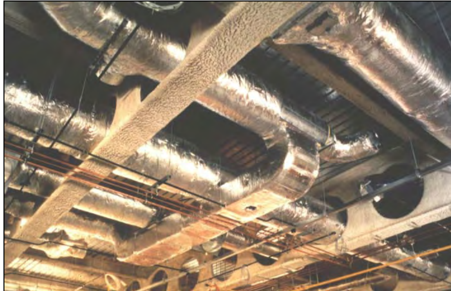
Figure 1.3 Services integrated with a cellular floor beam
