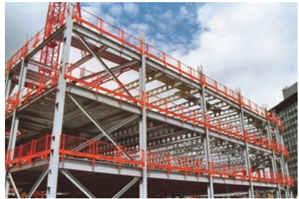
Steelwork ready for handover
