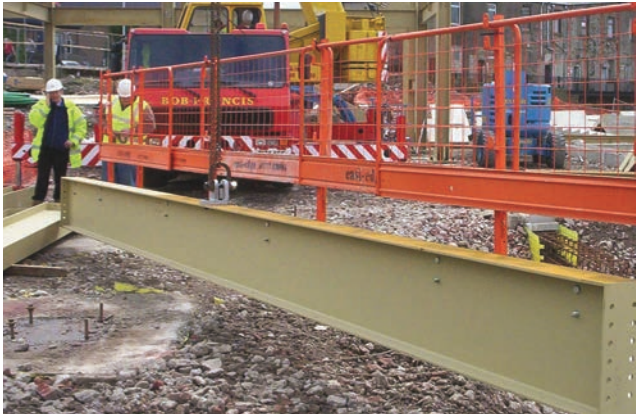
Use of the 'easi-edge' proprietary edge protection system
