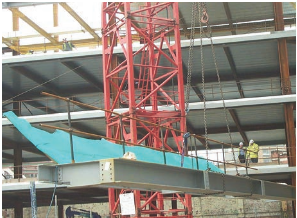
Debris netting fixed to perimeter beam before erection
