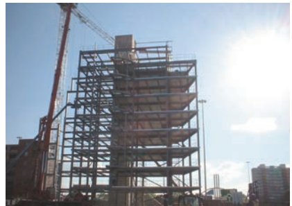
Multi-storey erection can use 35m MEWPs that reach the eighth level
