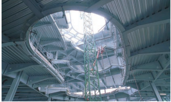
Tower crane located centrally within atrium
