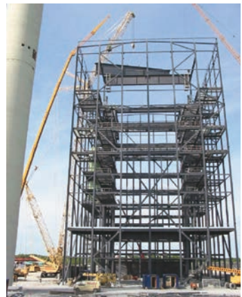
Scaffolded working positions attached to high level beams before erection
