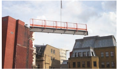
Beam dressed with 'easi-edge' protection
