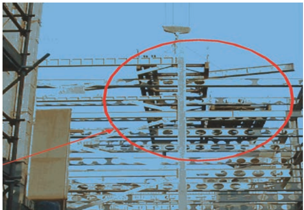
High level storage platform located onto the steelwork for use where there is insufficient storage at ground level
