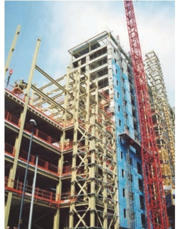
MEWP operating over slab
