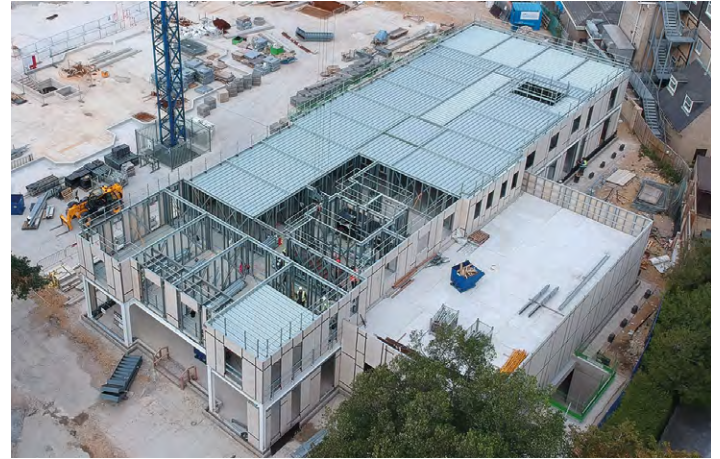
Figure 2: Light steel frame construction with metal decking for composite floors
