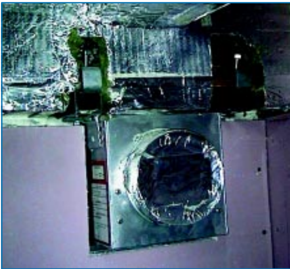
Figure 13: A fire damper suspended from a beam. Poor co-ordination forced the cutting of the beam fire protection system for Unistrut fixings – a typical improvisation by a services installer.
