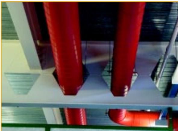
Figure 4: A typical castellated beam assembly, formed by cutting and re-welding standard universal beams. ©The Steel Construction Institute.
