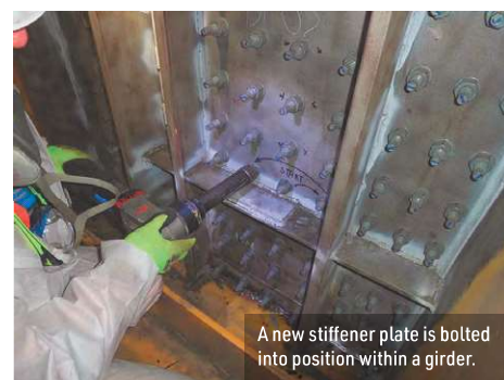
One of the original welded connections is repaired by the Taziker team.
