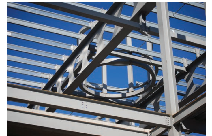
Circular openings over the pool areas rise above roof deck level
