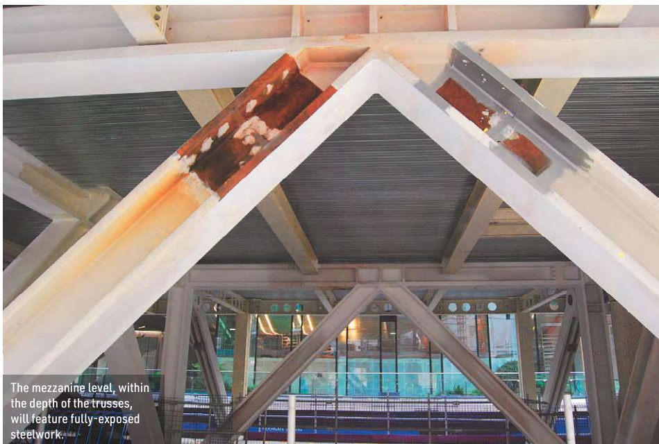
A series of trusses span London Underground assets and support the building's upper levels.
