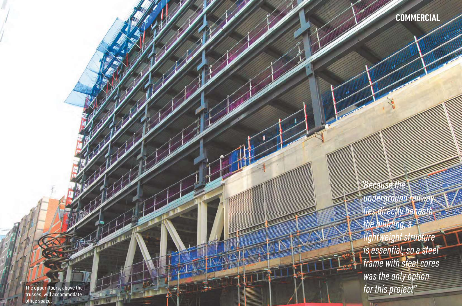
A series of trusses span London Underground assets and support the building's upper levels.
