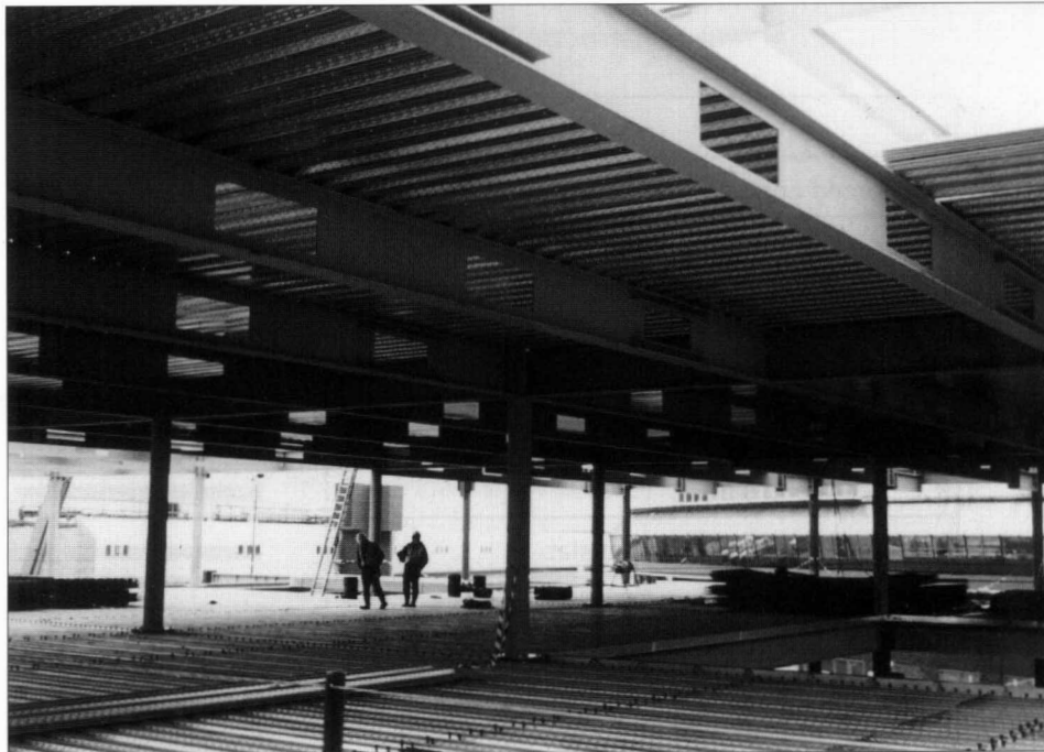
Figure 19 Openings in the webs of composite beams
