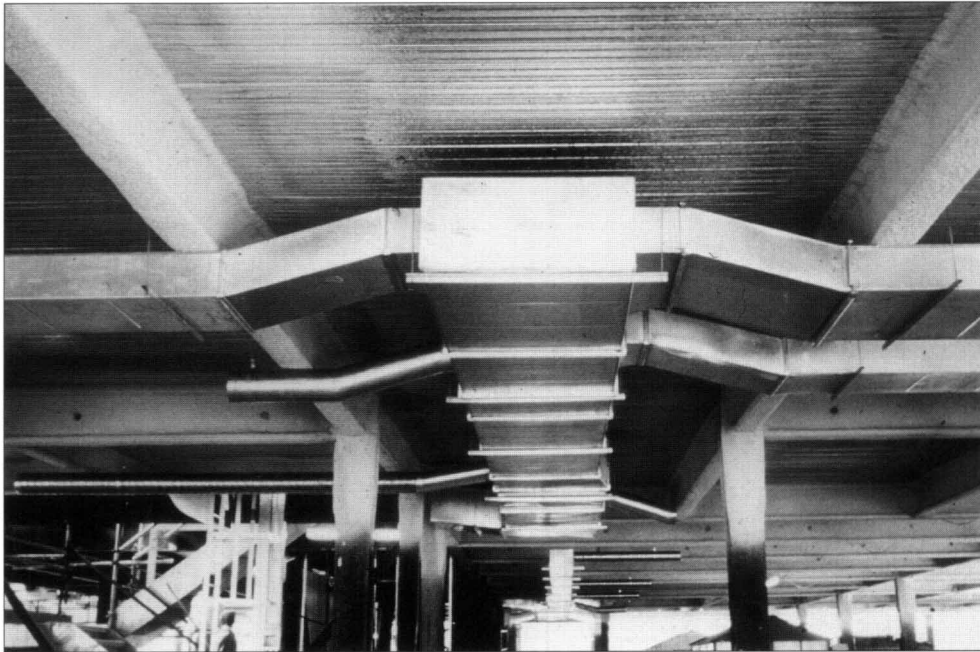
Figure 3 Example of partial services integration
