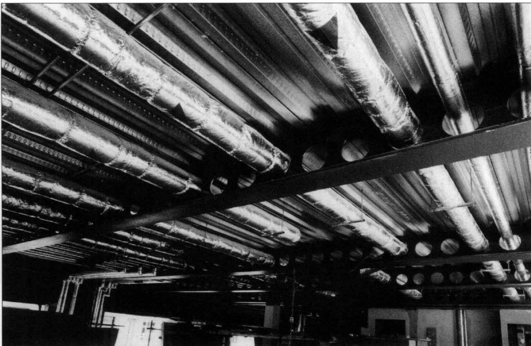
Figure 21 Cellular beam showing distribution of circular ducts
