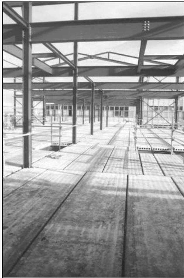
Figure 5.17 Precast concrete units on steelwork
