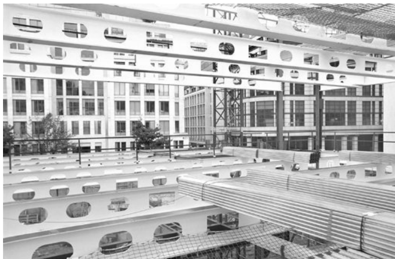
Figure 5.9 Fabricated beam with off-site fire protection
