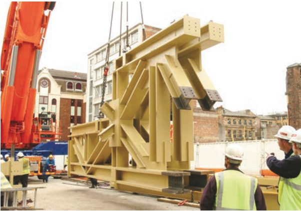
Truss lifted by counterbalanced crane
