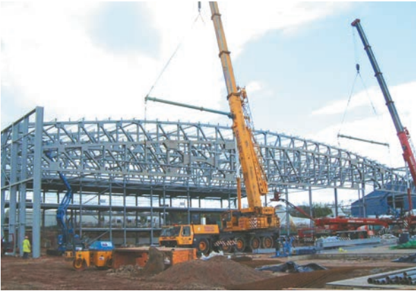
Tandem Lift using matched cranes
