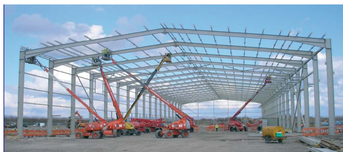
Figure 6: Portal frame with thoughtfully spaced purlins
