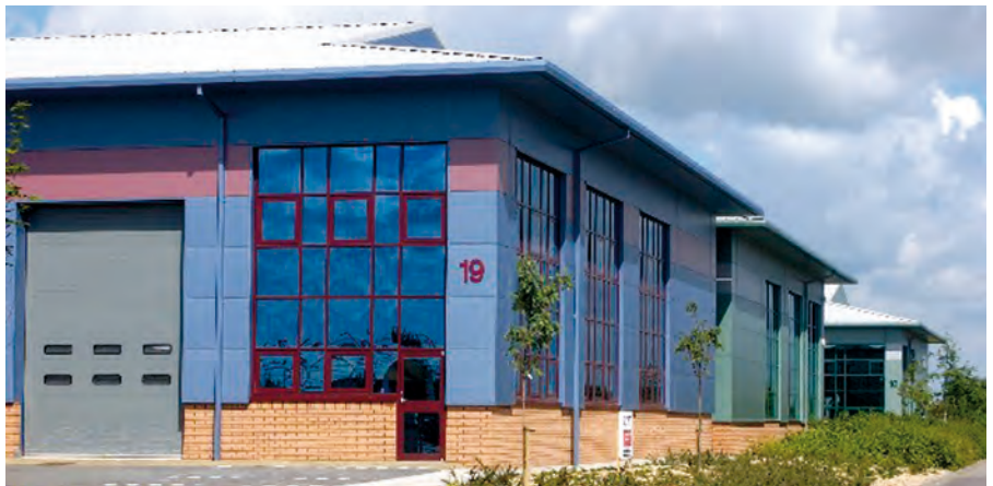
Figure 4.11 Large window and composite panels with 'dado' brick wall
