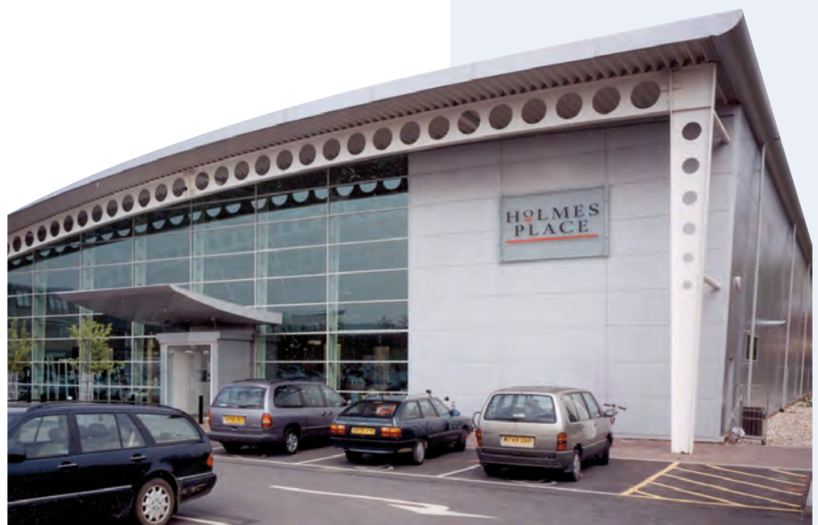
Figure 1.1 Leisure building using a steel framed structure
