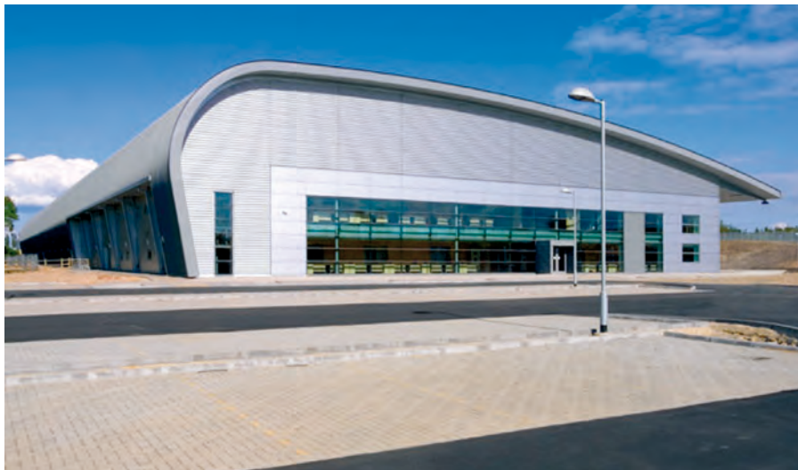
Figure 5.19 Curved steel sections used in a modern industrial building in the UK
