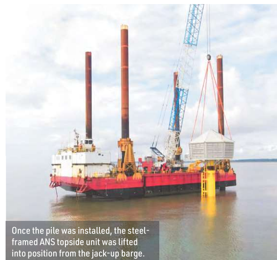
An assembled topside unit is lifted on to the barge.
