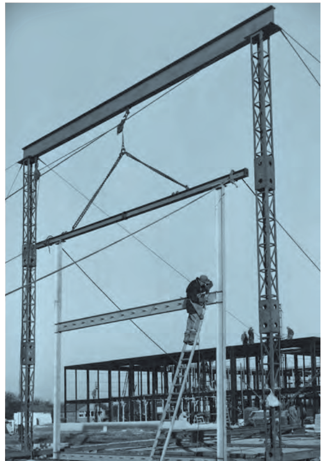
Right Slim beams and girders go up during the construction of Hunstanton School.
