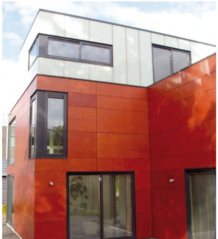
Figure 8.9 (Above & right) Smart House, Rotterdam using Square & Rectangular Hollow Sections with light steel infill walls & floor joists
