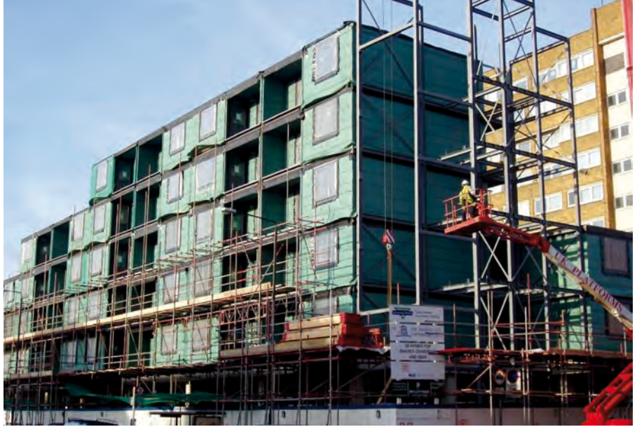
Figure 6.6 Modular building supported on a podium level and stabilised by a braced steel structure around the stairs
