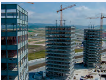
Bioclimatic Towers under construction
