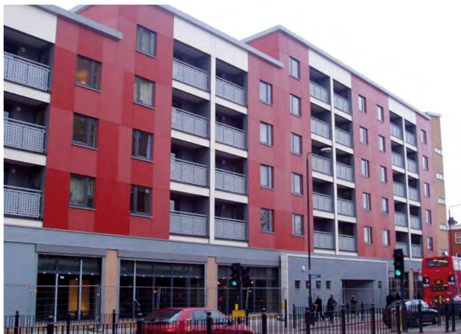
Figure 6.7 Completed modular building in Figure 6.6
