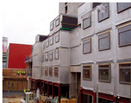
Installation of module on steel podium
