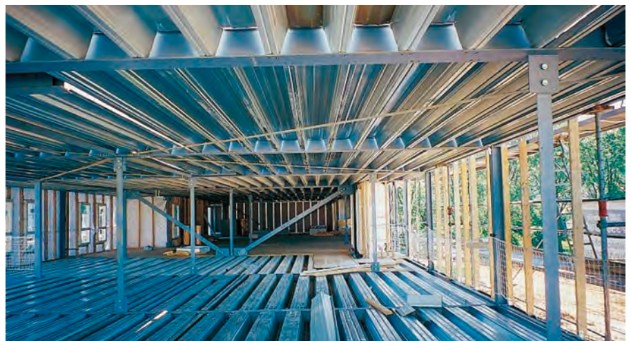
(Right) Intermediate floor showing wide open space for flexible arrangement of partitions and intensive use of steel elements
