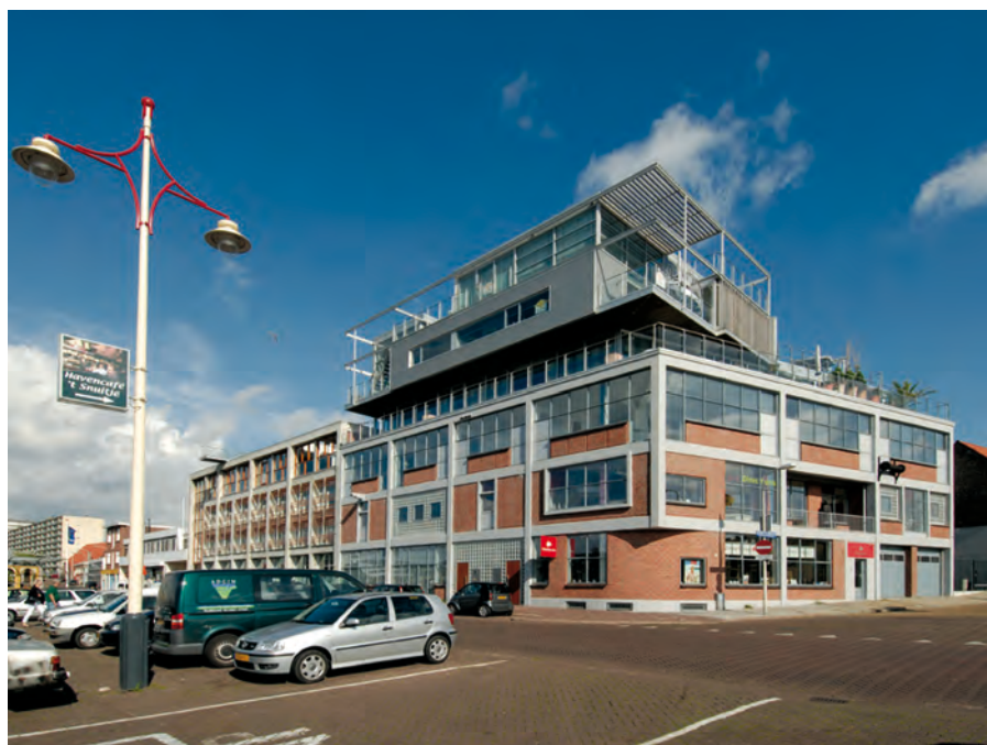
Figure 8.6 Transformation of an old warehouse with a spectacular view: Nautilus & IJsviss in The Hague (Winner National Steel Prize 2006, category Residential buildings).
