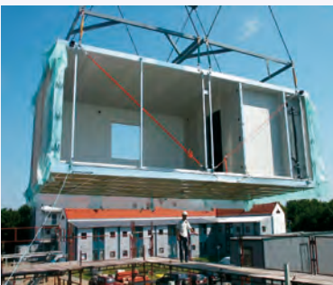
OpenHouse module during installation showing use of open sided modules with additional temporary posts
