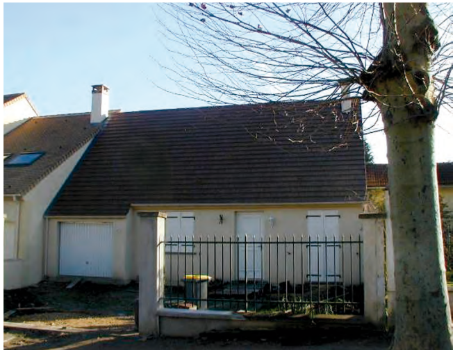
Figure 8.14 Maison Phénix during construction, showing the roof details for a single storey house
