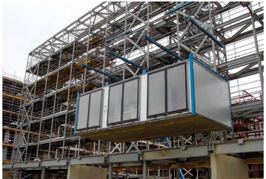
Figure 8.3 Steel external framework combined with highly glazed modules, MOHO, Manchester Yorkon and Shed KM Architects
