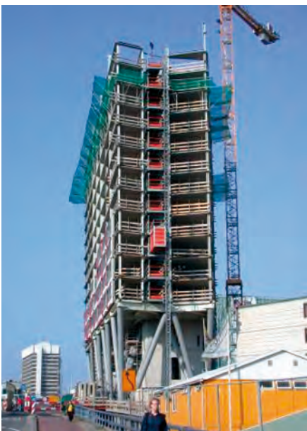
(Above) Building during construction
