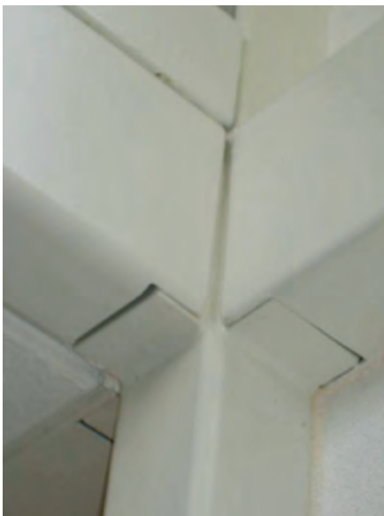
Figure 8.8 Town houses: House De Kom in Oranjewoud.
