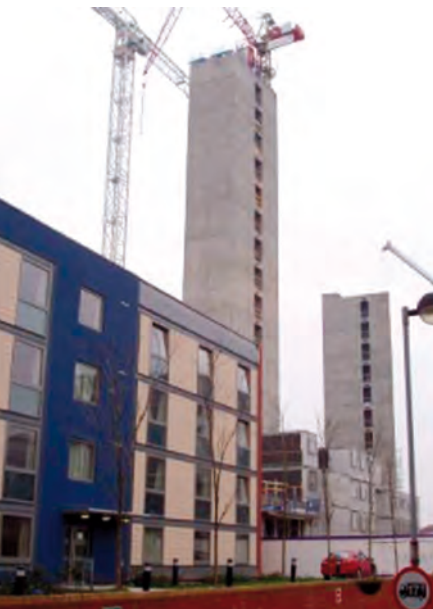
Modules attached to concrete core
