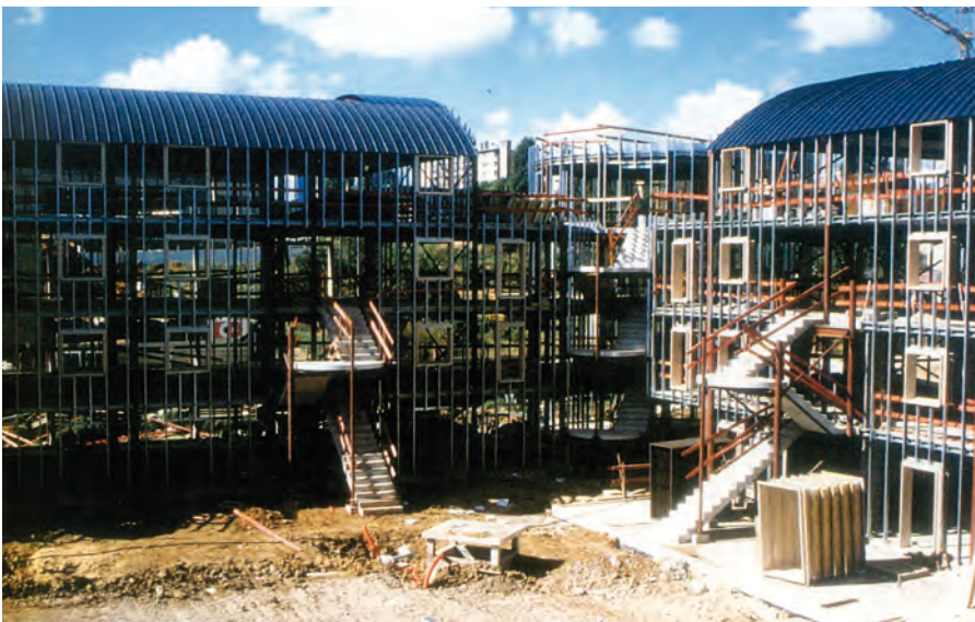
Figure 8.10 The PRISM system during construction: Steel frame, roof and external light steel walls ready to receive external skin
