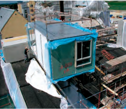
(Above) Module installation and completed façades
