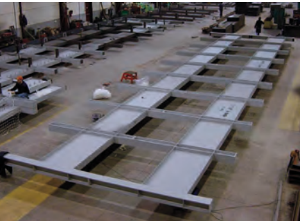
Off-site fabrication of the façade structural panels
