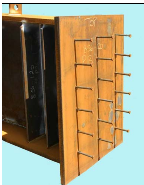
Figure 9.10 End plate of main girder, for connection to endscreen wall
