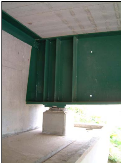
Overbridge on BNRR (Photo by SCI)
