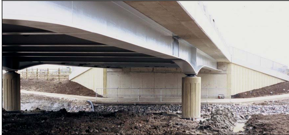
Semington Brook bridge (Photo by courtesy of Arup)
