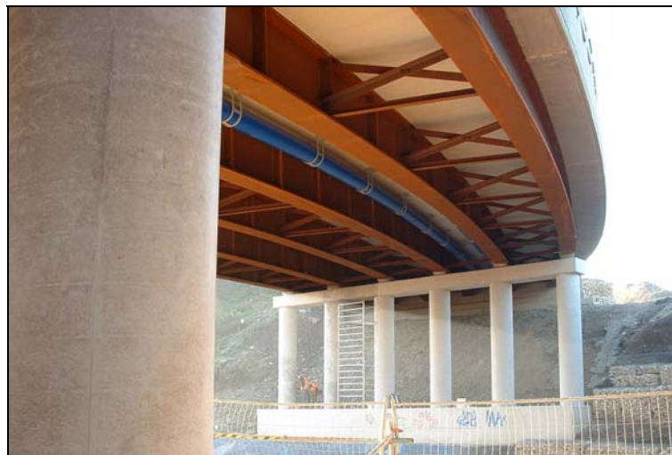
Highfield Lane Bridge (Photo by courtesy of Mabey Bridge)
