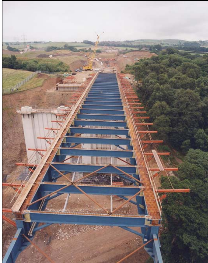
M65 Whitebirk viaduct (Photo by courtesy of Mabey Bridge)
