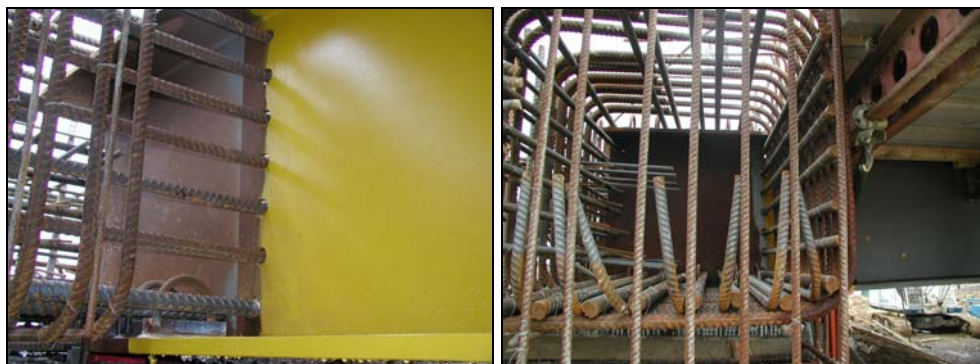
Figure 9.8 Reinforcement in endscreen wall
