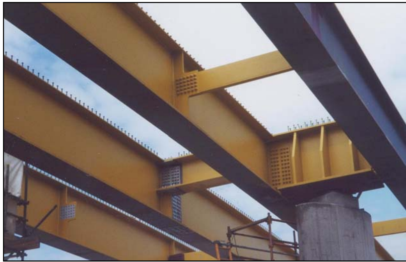
Overbridge on BNRR (Photo by courtesy of Mabey Bridge)
