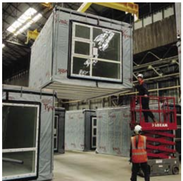
Semi-automated production line at Corus Living Solutions' factory.
