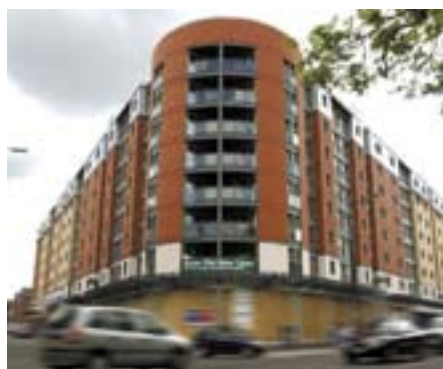
Modules supported on a steel podium at first floor. Courtesy, The Design Büro/Ayrshire Framing.
