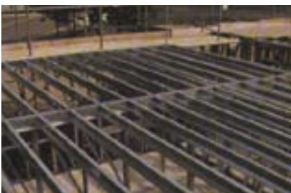
Floor joists, usually of C or Z sections that are placed individually or installed as pre-fabricated floor cassettes.
