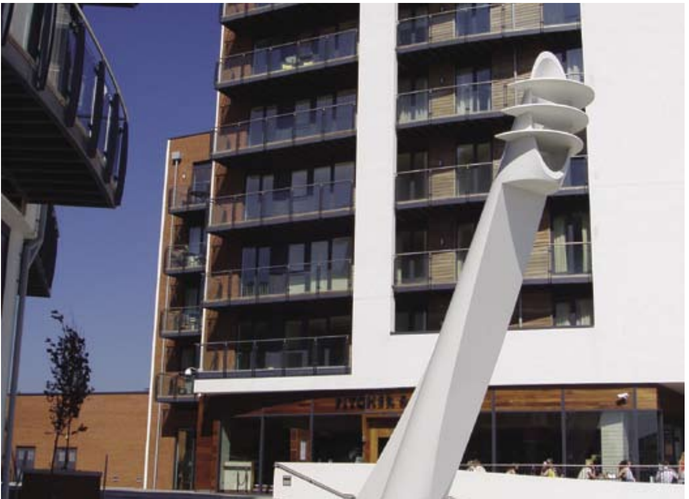
Ocean Village, Southampton: Multi-storey composite building with balconies. Courtesy, Broadway Malyan Architects.
