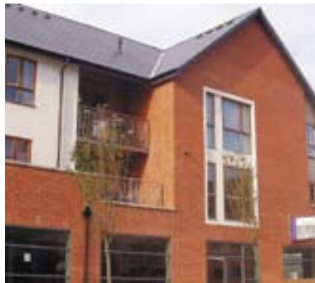
Apartments and shop using light steel framing. Courtesy, HTA Architects.
