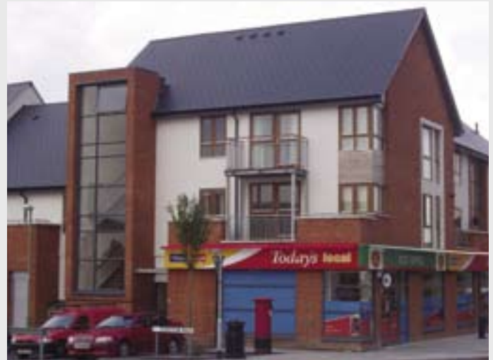
3-storey apartments and shop using light steel framing. Oakfern redevelopment, Basingstoke. Courtesy, HTA Architects.
