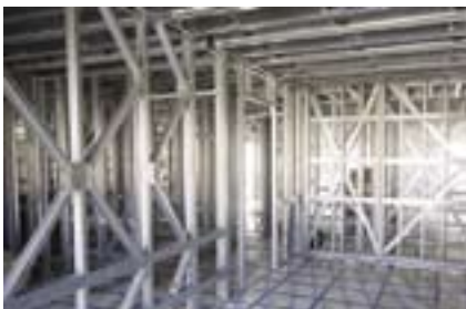
Load bearing wall panels. Courtesy, Framing Solutions.
