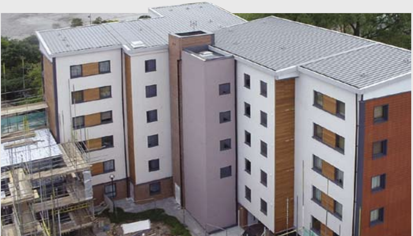
Apartments using load-bearing light steel frames. Courtesy, Framing Solutions.
