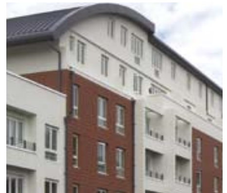
Light steel infill walls in a multi-storey apartment building. Courtesy, RDJW Architects.
