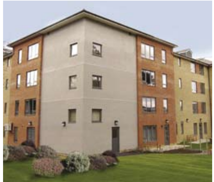
Apartments using light steel framing. Courtesy, Fusion Building Systems.
