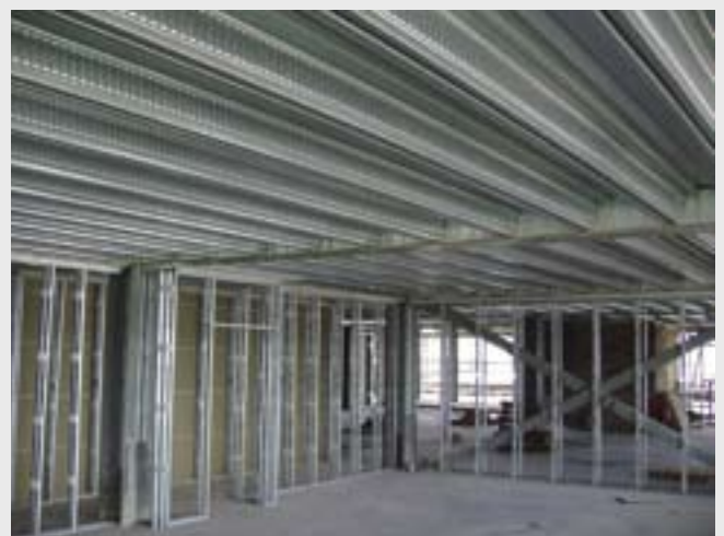
Slimdek structure with light steel infill walls.
