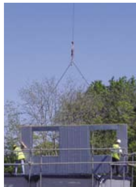
Courtesy, Fusion Building Systems.
