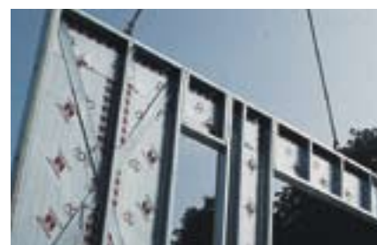
Prefabricated load-bearing wall panels using C sections.
