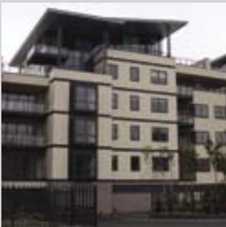
Courtesy, Fusion Building Systems.
