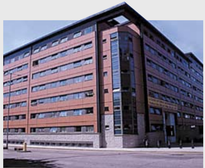
Modular student accommodation, Manchester. Courtesy, The Design Büro, Caledonian Building Systems.
