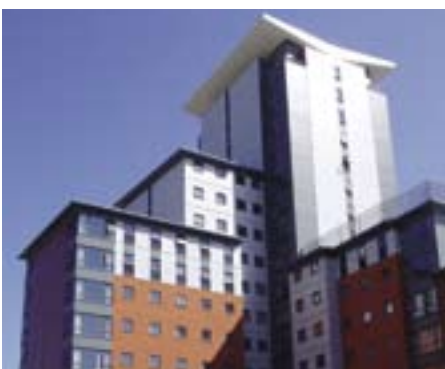
Steel framework for multi-storey apartments. Courtesy, Unite Modular Solutions.
