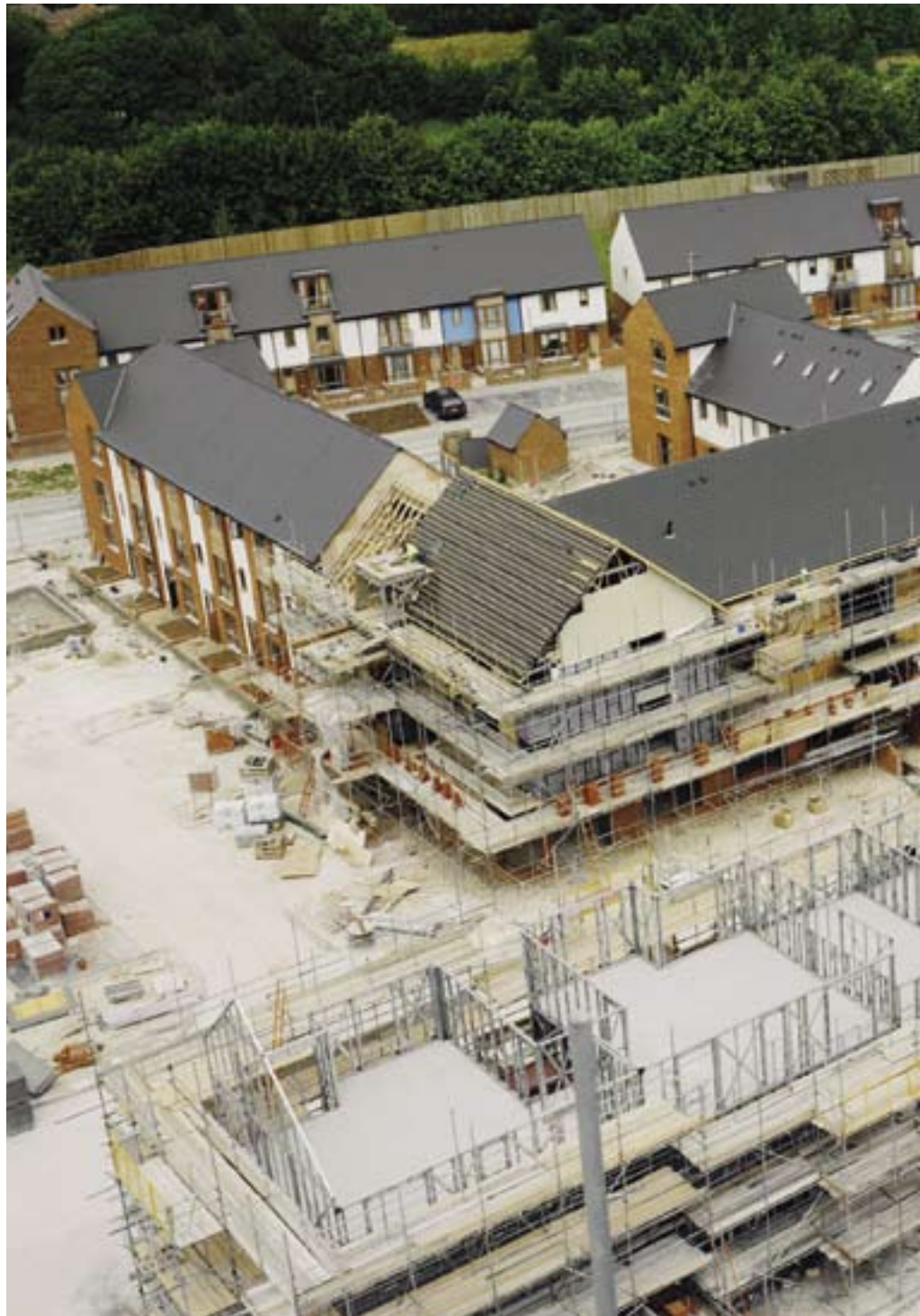
Light steel framing during construction. Oakfern redevelopment, Basingstoke. Courtesy, HTA Architects.
