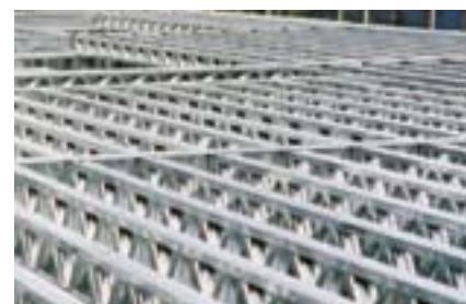
Lattice joists used for longer spans.
