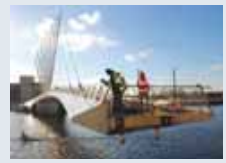
The steel construction means the deck can be very thin.
