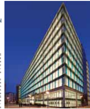
air-conditioning system was considered but at the time this wasn't widely accepted by clients and investors and so was not used.
