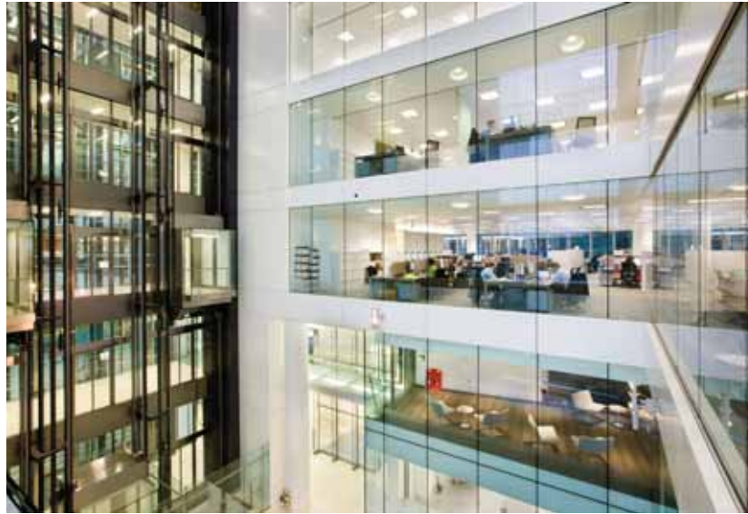
One Kingdom Street is designed around two central atriums, which help reduce solar gain.
