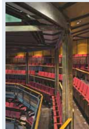
Steelwork in the auditorium was left untreated for a raw finish.
