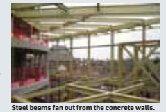
Steel beams fan out from the concrete walls.
