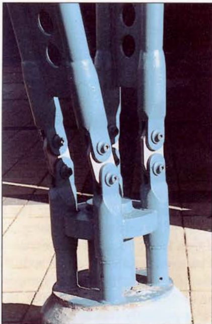
Figure 1.2 Cast fork-end connectors in the Clydebank Tourist Village
