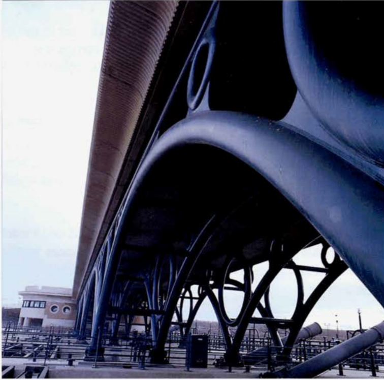
Circular infill casting
