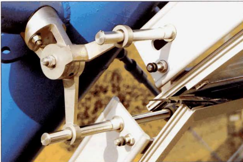
Stainless steel glazing connection
