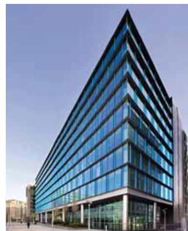
Test showed that less carbon was produced as a result of the decision to use a steel frame on One Kingdom Street in London
