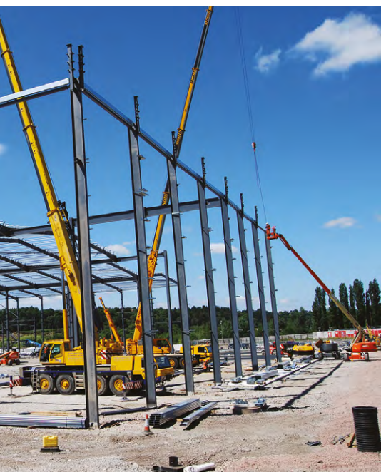
Steelwork erection progresses on the four-span portal-framed structure.
