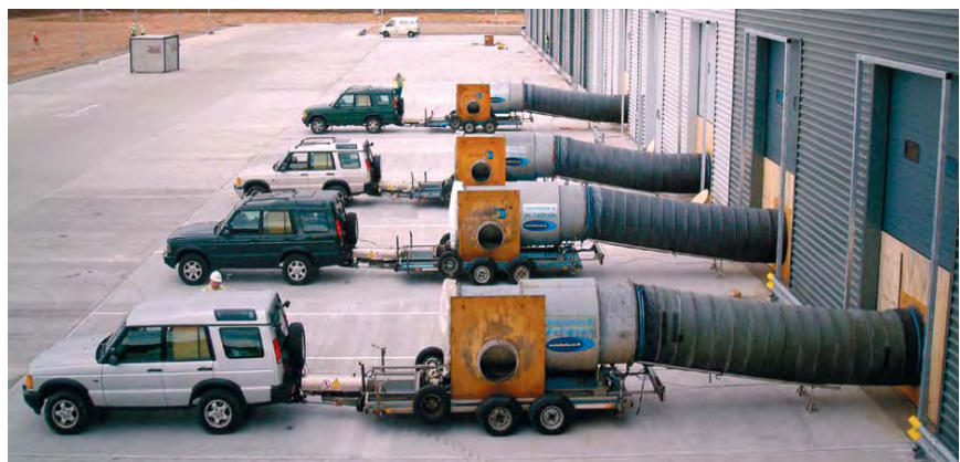
Pressure testing at the B&Q Distribution Centre, Worksp Courtesy of BSRIA
