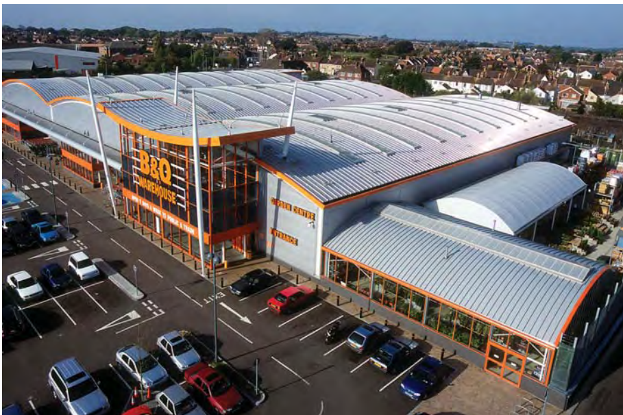
B & Q, Ashford Courtesy of C A Roofing
