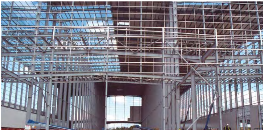
Construction of the steel frame Courtesy of Billington Structures Ltd.
