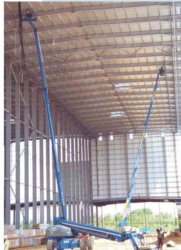
Use of mobile access platforms Courtesy of Billington Structures Ltd
