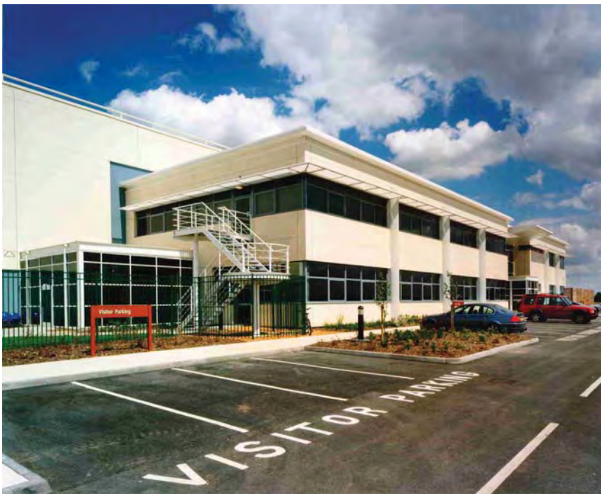
Office adjoining a large distribution warehouse Courtesy of Hathaway Roofing
