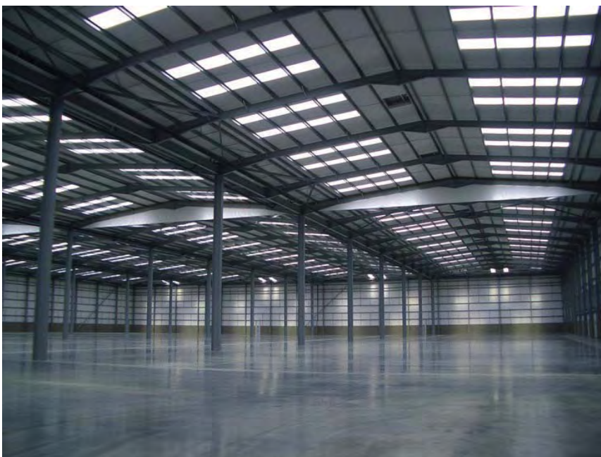
Typical rooflight pattern in an industrial shed Courtesy of Caunton Engineering Ltd.
