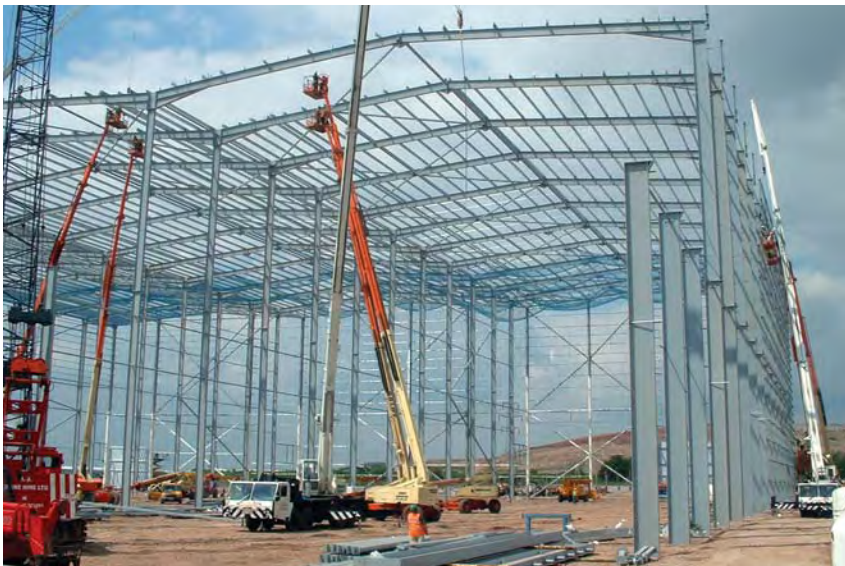
Kingswood Lakeside Business Park, Cannock Courtesy of Barrett Steel Buildings Ltd.
