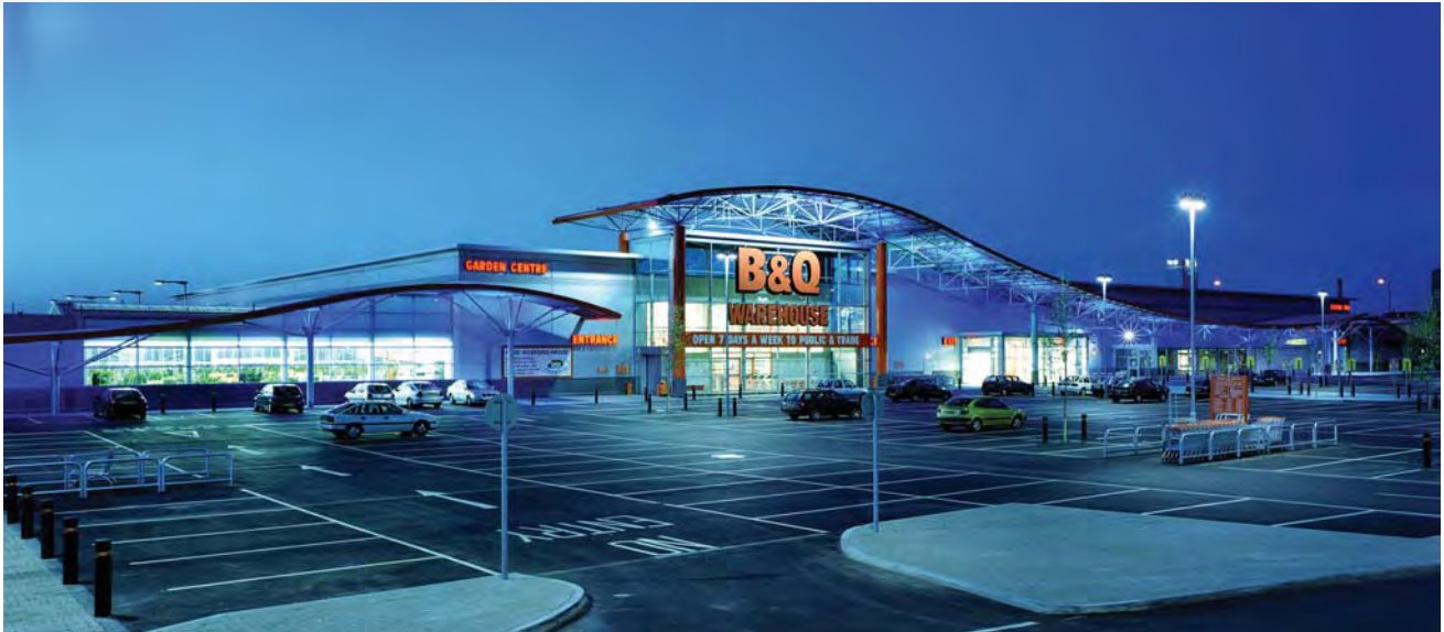
B&Q, Belvedere Courtesy of C A Roofing
