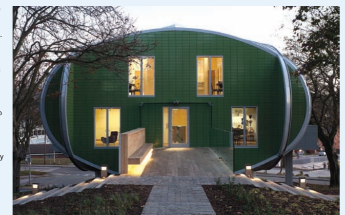
Entrance: each elevation is framed in an oval of steel.
