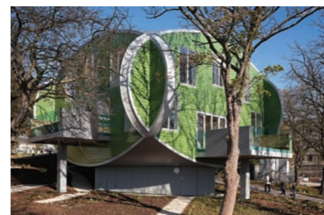
The structure gives the impression of floating on a pedestal.
