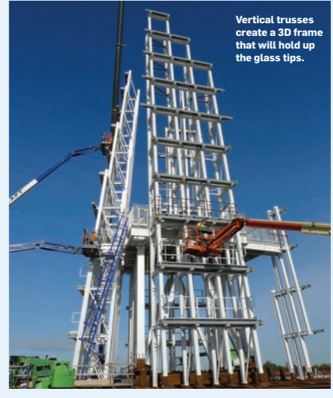
During the trial assembly, the spire was erected in three sections at Severfield-Reeve's Dalton plant.
