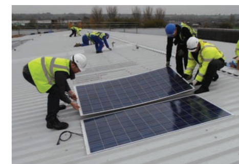
A frameless crystalline solar system was installed directly on to the Deeside Leisure Centre's metal roof.
