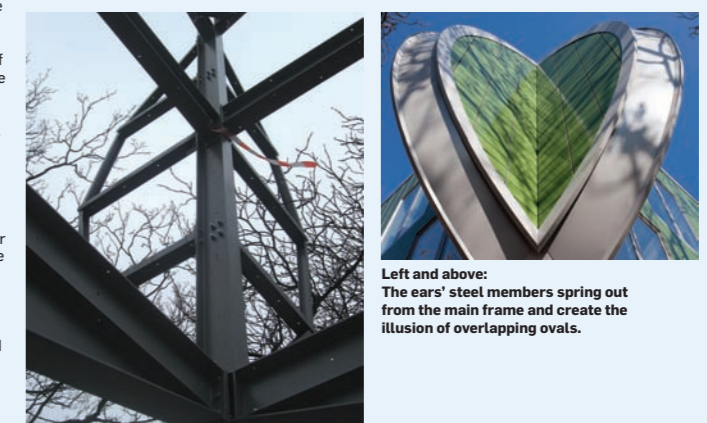
Entrance: each elevation is framed in an oval of steel.
