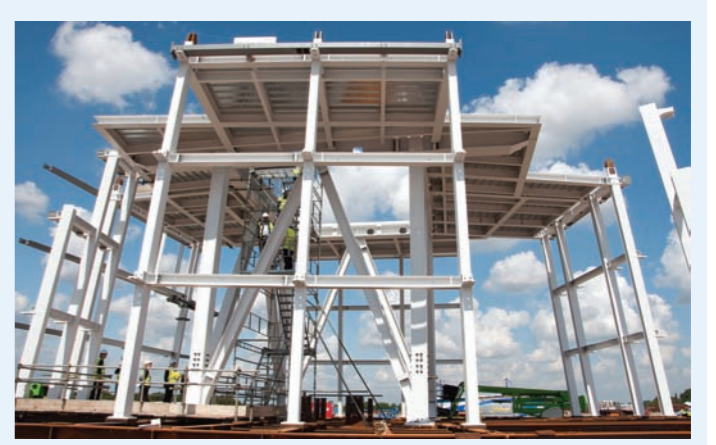
During the trial assembly, the spire was erected in three sections at Severfield-Reeve's Dalton plant.
